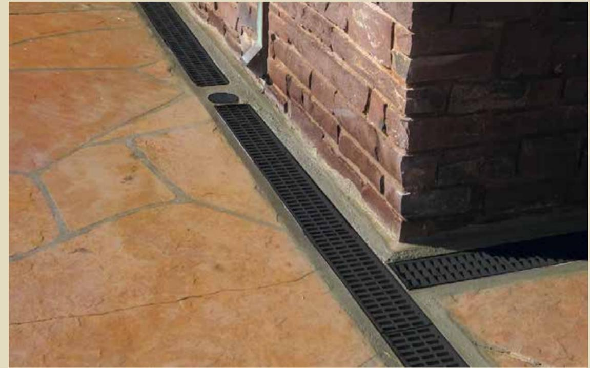
The surface channel that are used at present are of cast iron or in concrete and due to their heavy weight it is difficult to handle or storage or to install and more over they are prone to corrosion. ASTRAL offers surface channel made from polypropylene and they are free from above problems caused by traditional surface channel.
