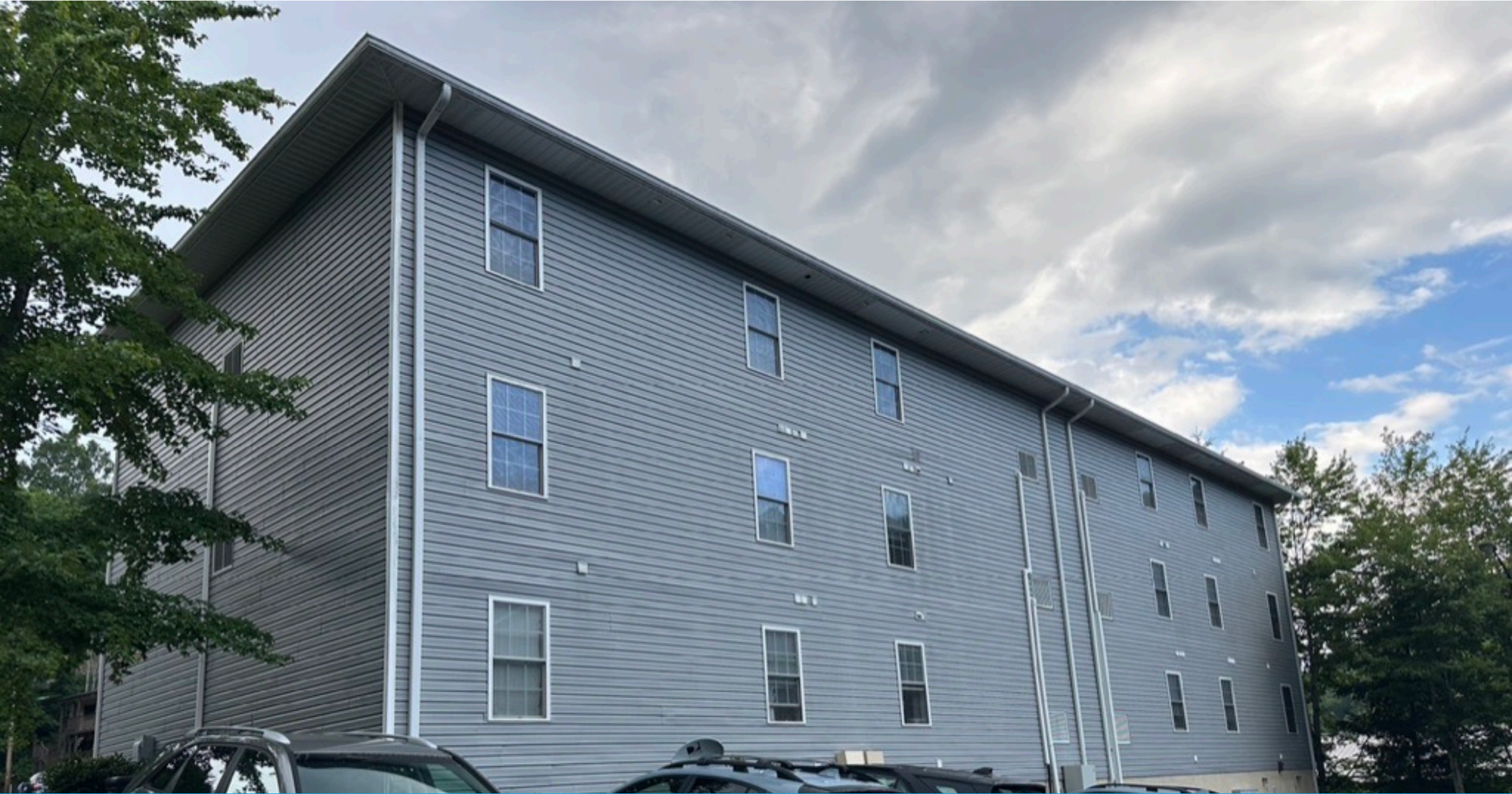
1555 West King Street | Side and Back of Building
