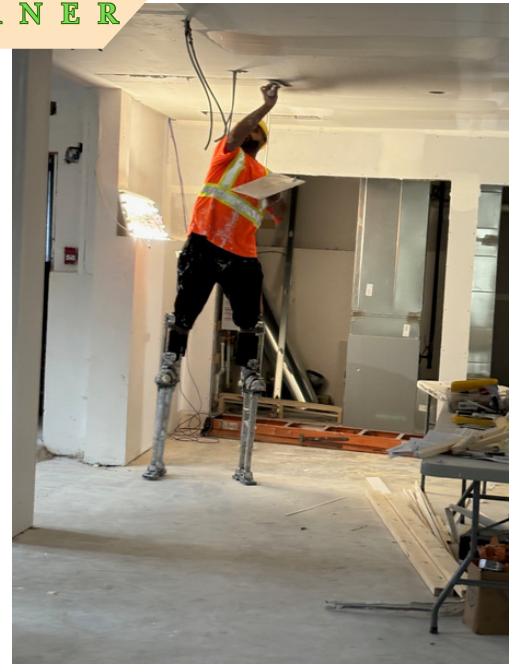
Drywallers on stilts: Getting ready for finishing.
