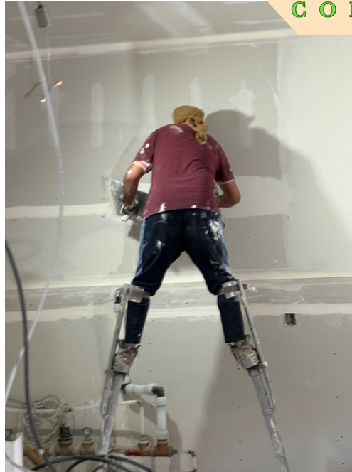
Drywallers on stilts: Getting ready for finishing.
