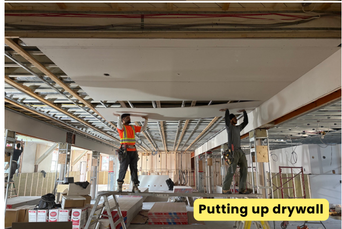
Putting up drywall
