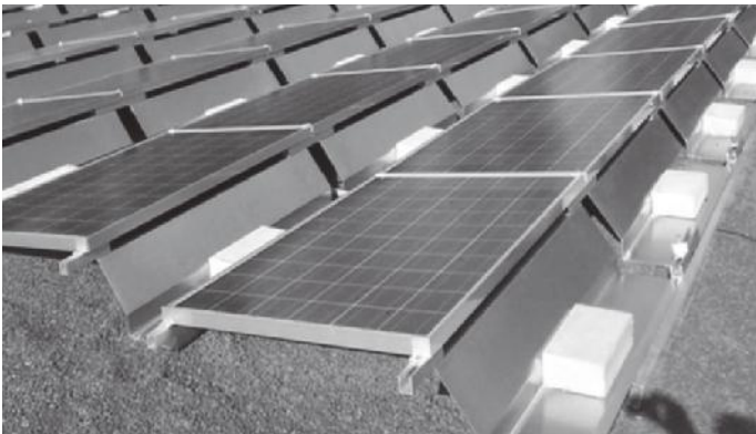
Figure 9.3 Ballasted system Source: Courtesy Advanced Solar Products, Solstice Mounting System.
