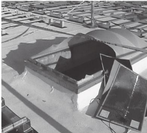
The skylight that the worker fell through
