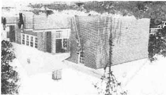
Destroyed by Fire
