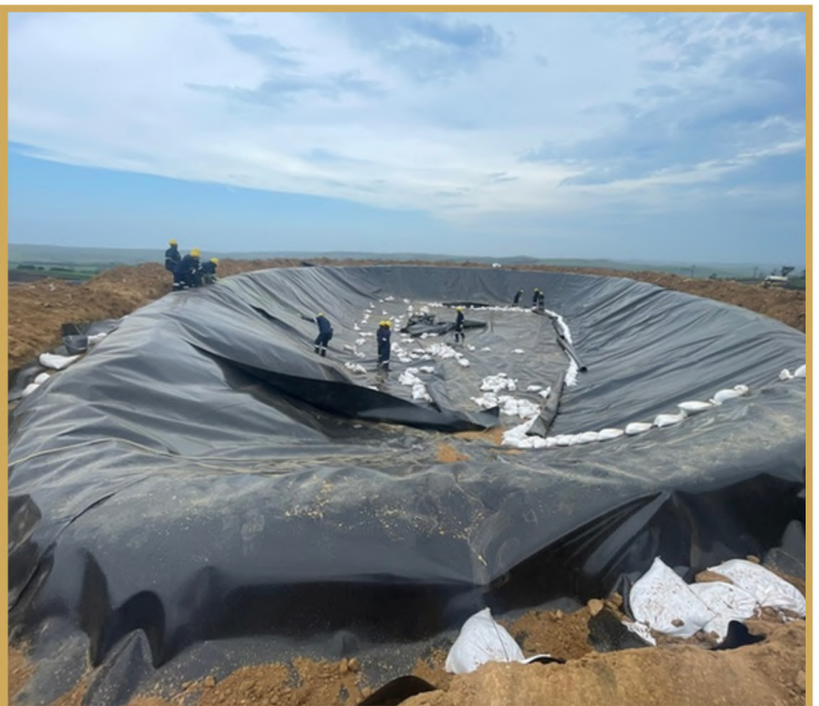
Installation of primary geomembrane and secondary geomembrane (floating cover) on the leachate pond
