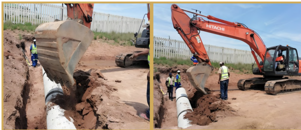
Bulk earthworks and installation of stormwater services
