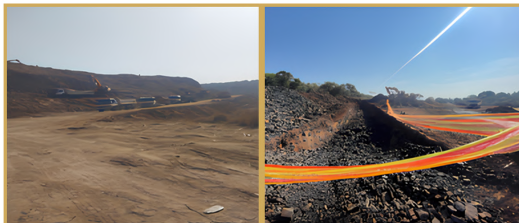
Bulk Earthworks – Borrow materials from the borrow pit, cut to spoil the road footprint
