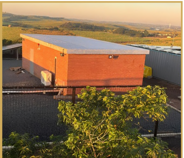
completed inverter building
