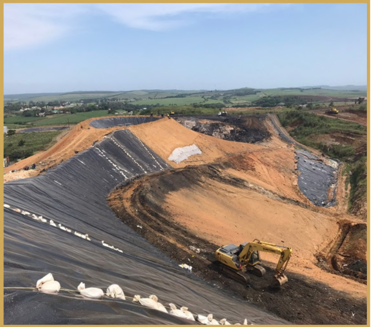
Bulk earthworks for leachate pond
