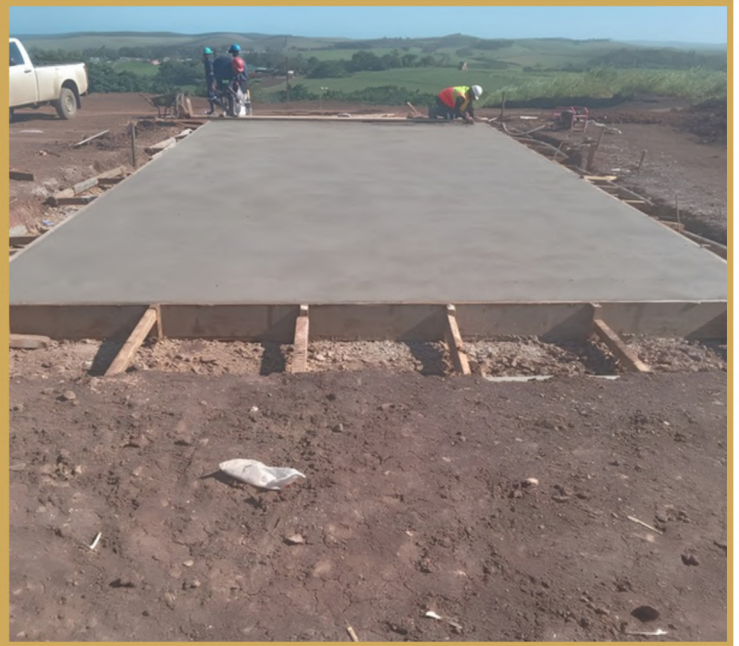
Earthworks and foundation slab for inverter building
