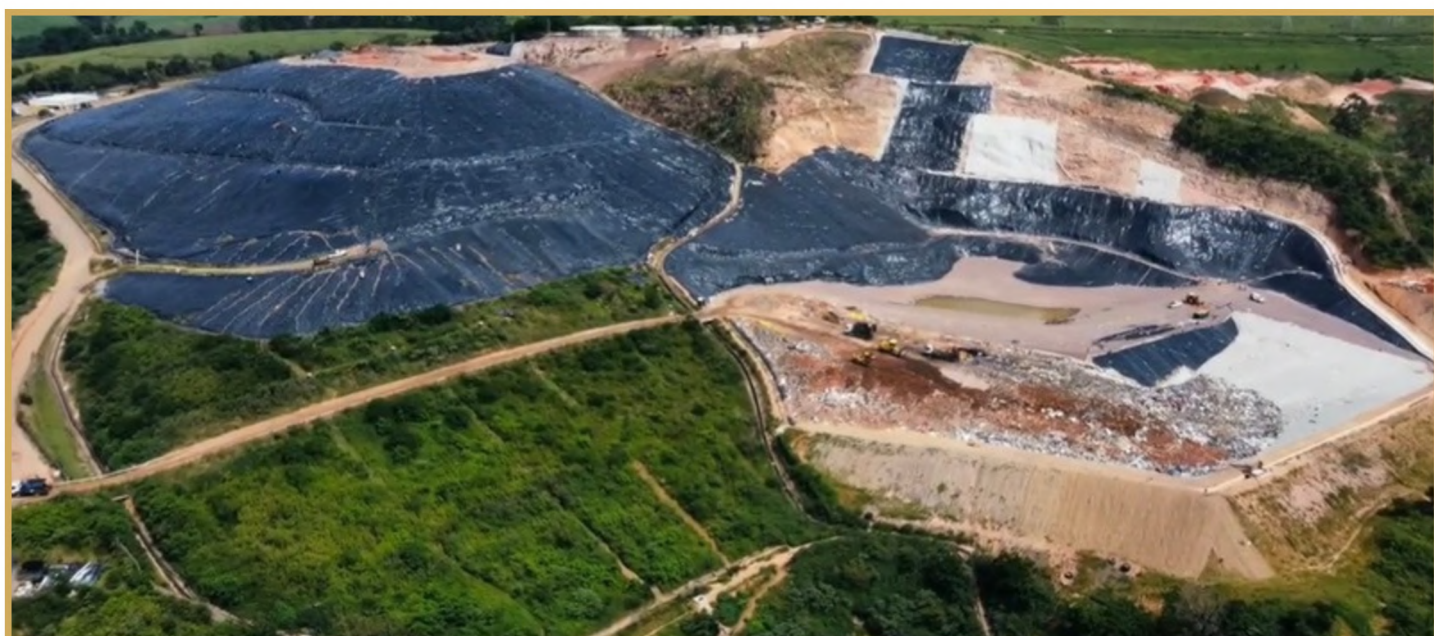
Completed Landfill Capping installed, including ballast layer and full stormwater drainage systems
