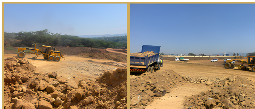
Tipping, levelling and compacting material from the borrow pit in fill
