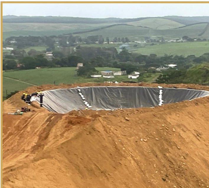
Installation of primary geomembrane and secondary geomembrane (floating cover) on the leachate pond
