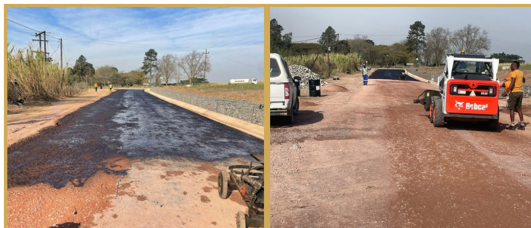
Layerworks, Priming Vdrains and Gabions
