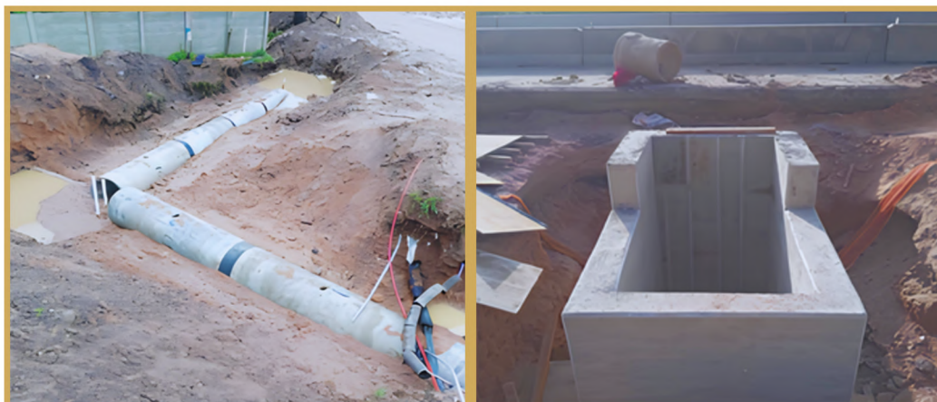
Installed stormwater pipeline, completed concrete stormwater inlet structure
