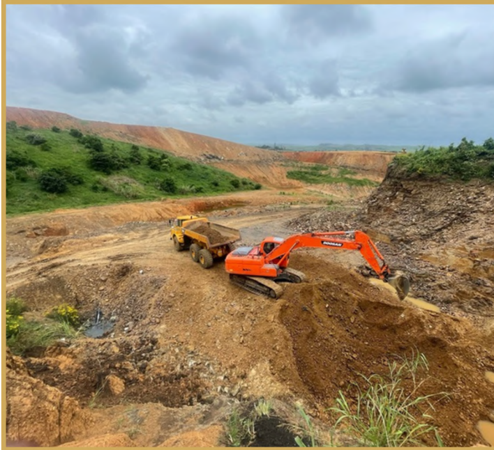
Bulk earthworks for leachate pond
