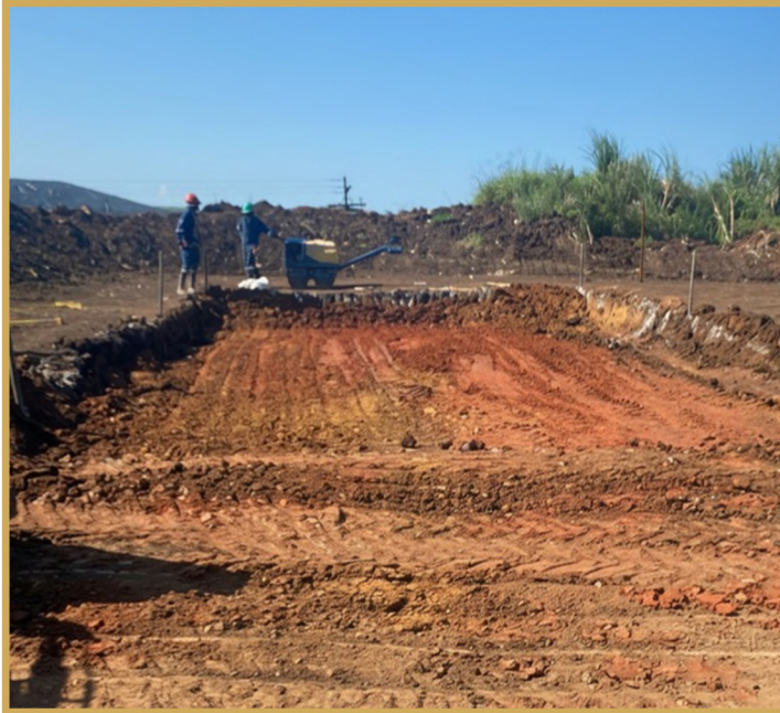
Earthworks and foundation slab for inverter building
