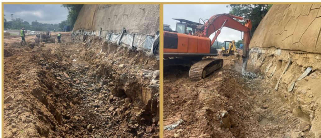
Excavation for stormwater lines, breaking rock on stormwater lines
