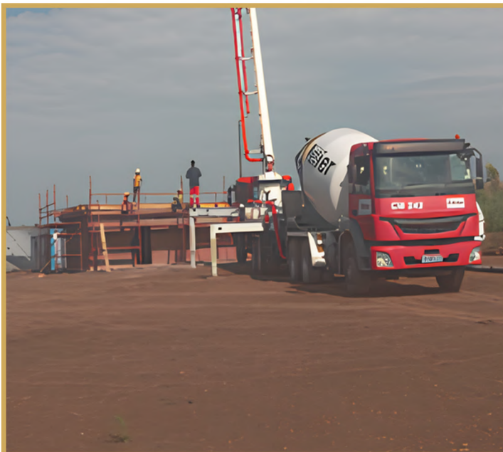
Casting the roof slab for the inverter building
