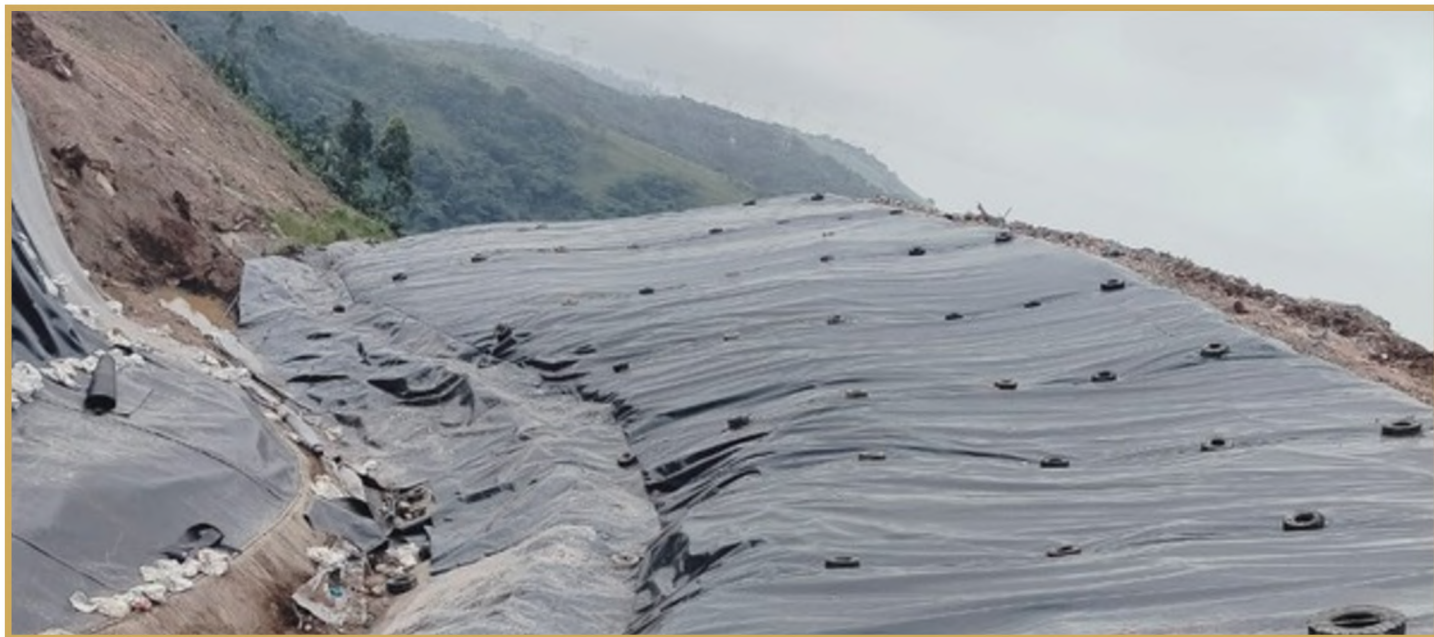
Completed Landfill Capping installed, including ballast layer and full stormwater drainage systems
