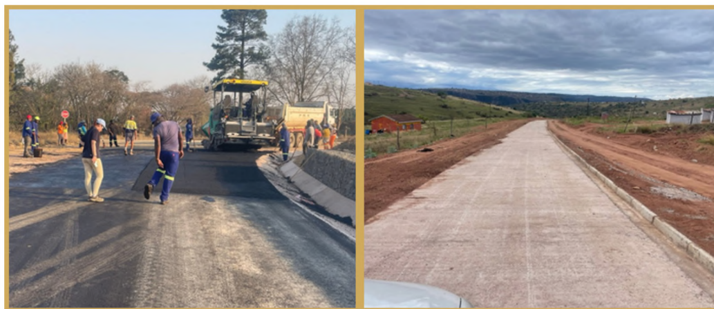
Completed asphalt and concrete pavement, including full service
