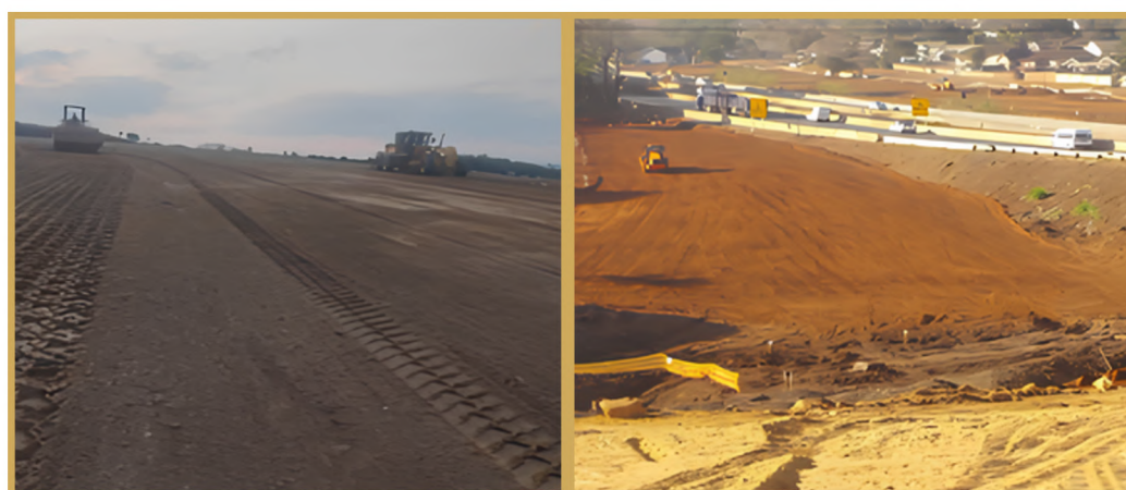
Bulk fill processed and completed
