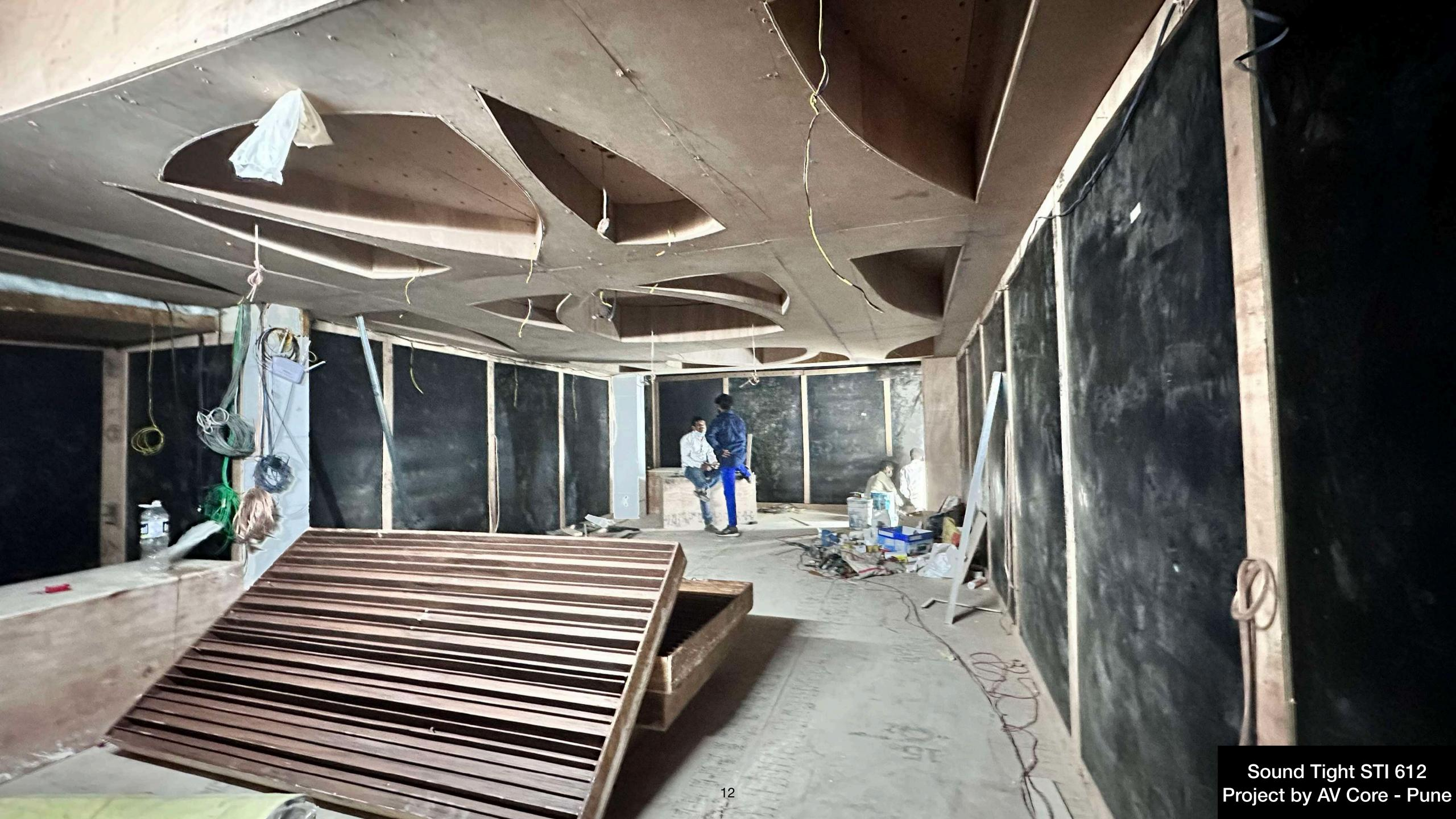
With STI 612 - 'Sound Tight' Elastomer, you can achieve very good sound isolation when applied in wall panelling.
