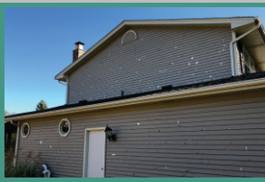
HAIL DAMAGED SIDING
