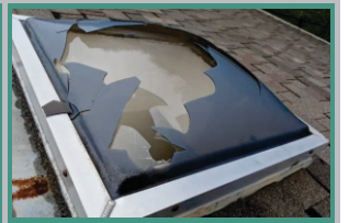
HAIL DAMAGED SKYLIGHTS
