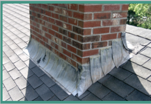
AGED CHIMNEY FLASHING
