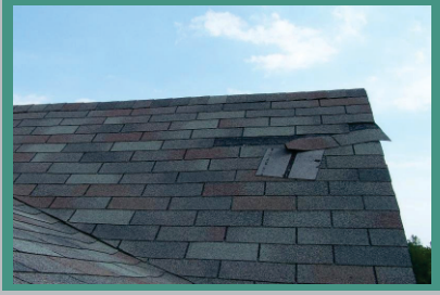
WIND DAMAGED SHINGLES
