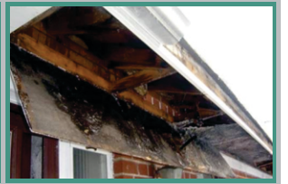
SOFFIT ROTTING
