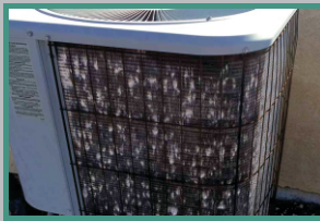
HAIL DAMAGED HVAC
