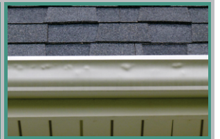
HAIL DAMAGED GUTTERS
