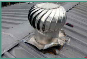
HAIL DAMAGED VENTS
