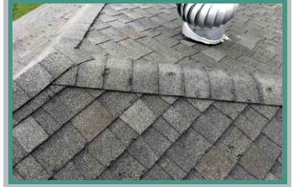
HAIL DAMAGED SHINGLES
