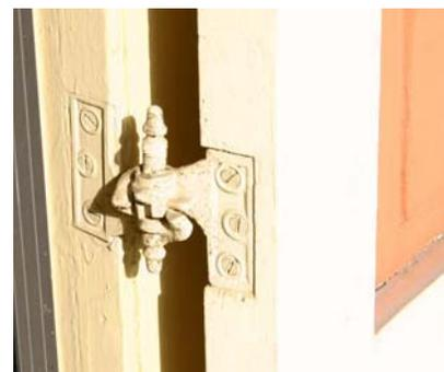
**CLARK'S TIP HINGES** are nearly identical in operation to Acme, Lull & Porter hinges but are surface-mounted.
