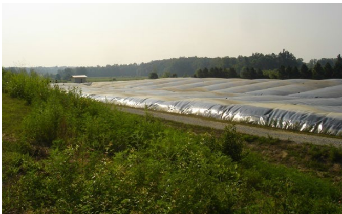
Covered lagoon where biogas from anaerobic digestion is captured. Reproduced with permission from Perdue Farms.
