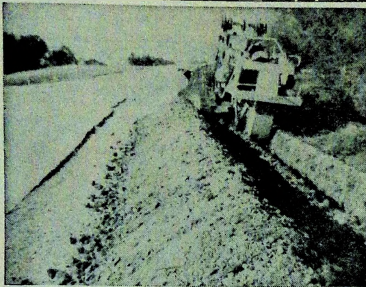
Trench is being dug for the gas lines to allow the City of Grey Forest to provide natural gas for residents of this area. Sub-surface of Fort Worth reports progress averaging a mile a day.
