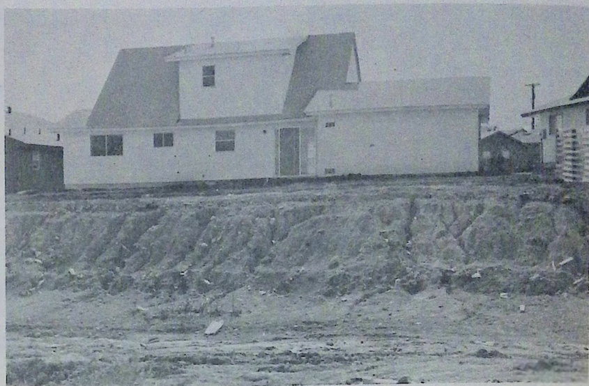
With the building boom predicted for this area, Soil Conservation experts warn developers and new home owners to avoid this type of erosion in new sub-divisions. Fortunately the soil here favors building, but some areas will require retaining walls, etc., developers have been told.
