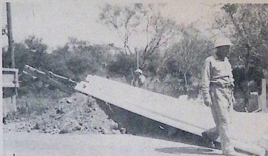
A worker checks some more conduits that will soon be added to the others going into the ground.
