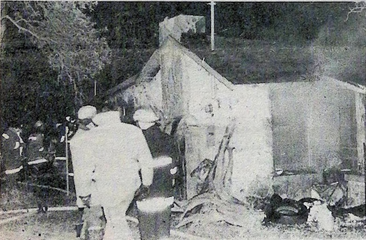
A fire that began about 9 o'clock on the chilly evening of Dec. 28 gutted the home of Peggy Sassaman, Grey Forest city council member, at the corner of Bluebonnet Drive and Park Drive. The fire reportedly started in a wall furnace.
