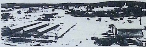
The 3,500-watt (peak) solar cell array field (left foreground) is the main element of the world's first solar electric village power system.
