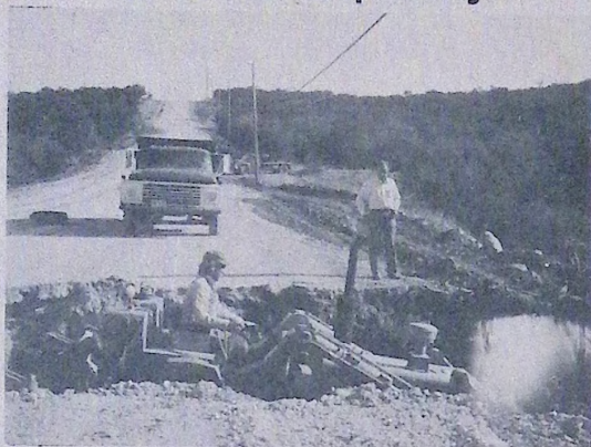
Here, workers employed by Border Asphalt Co. dig a trench where a culvert will be added to meet drainage specifications. This is Cross XD Trail which links Bar X Trail with Scenic Loop Road.
