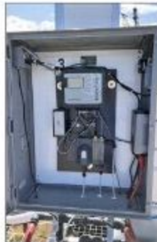
The farming operation's new treatment system includes sensors for real-time monitoring and management of chlorine, pH levels and temperature in surface sourced irrigation water. (Submitted photo)
