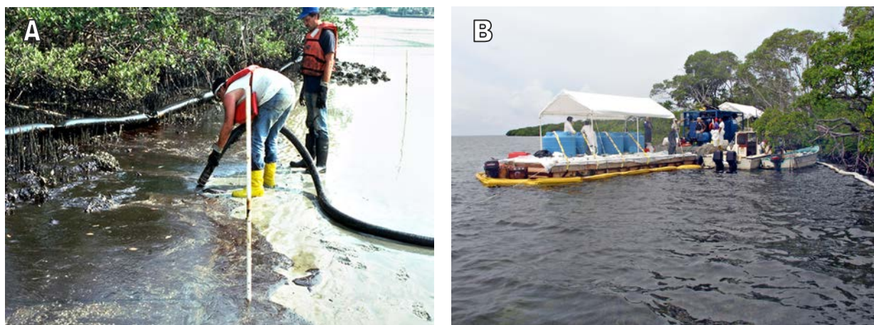
Figure 3.4. Vacuuming techniques in mangroves. A) Successful removal of thick oil from mangroves working on a firm sand flat during the 1993 Tampa Bay, Florida spill (Jacqueline Michel, Research Planning, Inc.) B) Unsuccessful attempt to remove floating oil trapped in the mangrove fringe during the 2007 Guánica, Puerto Rico spill of heavy fuel oil. Note the multiple tanks to separate the large volume of water recovered (Brad Benggio, NOAA).
