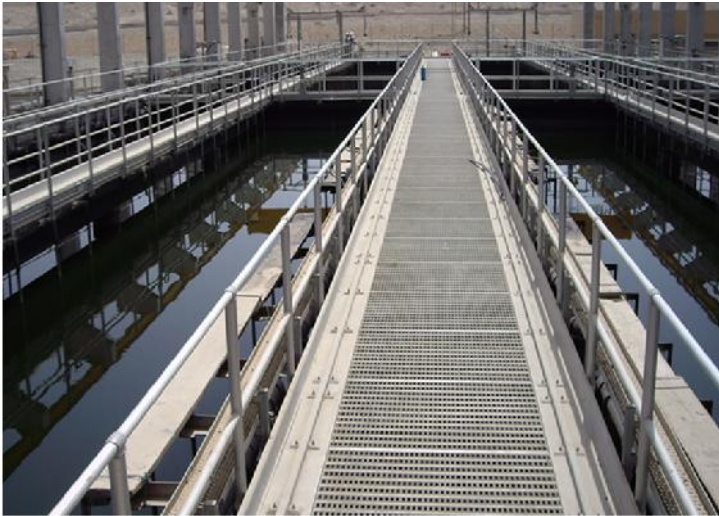
Aluminum Walkway and handrails installed in Water treatment facilities
