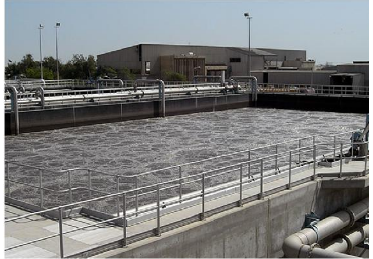
Aluminum Walkway and handrails installed in Water treatment facilities
