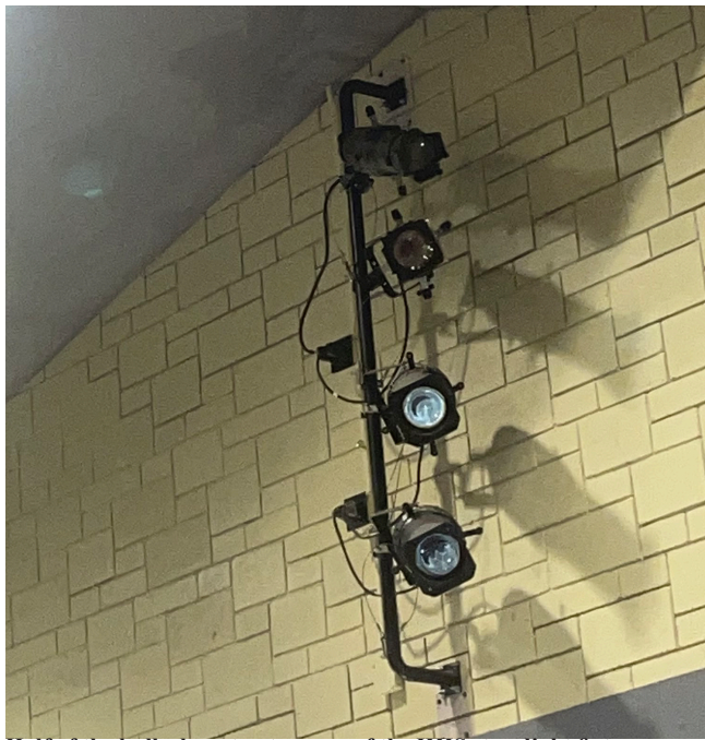
Half of the bulbs burnt out on one of the HHS stagelight fixtures.
