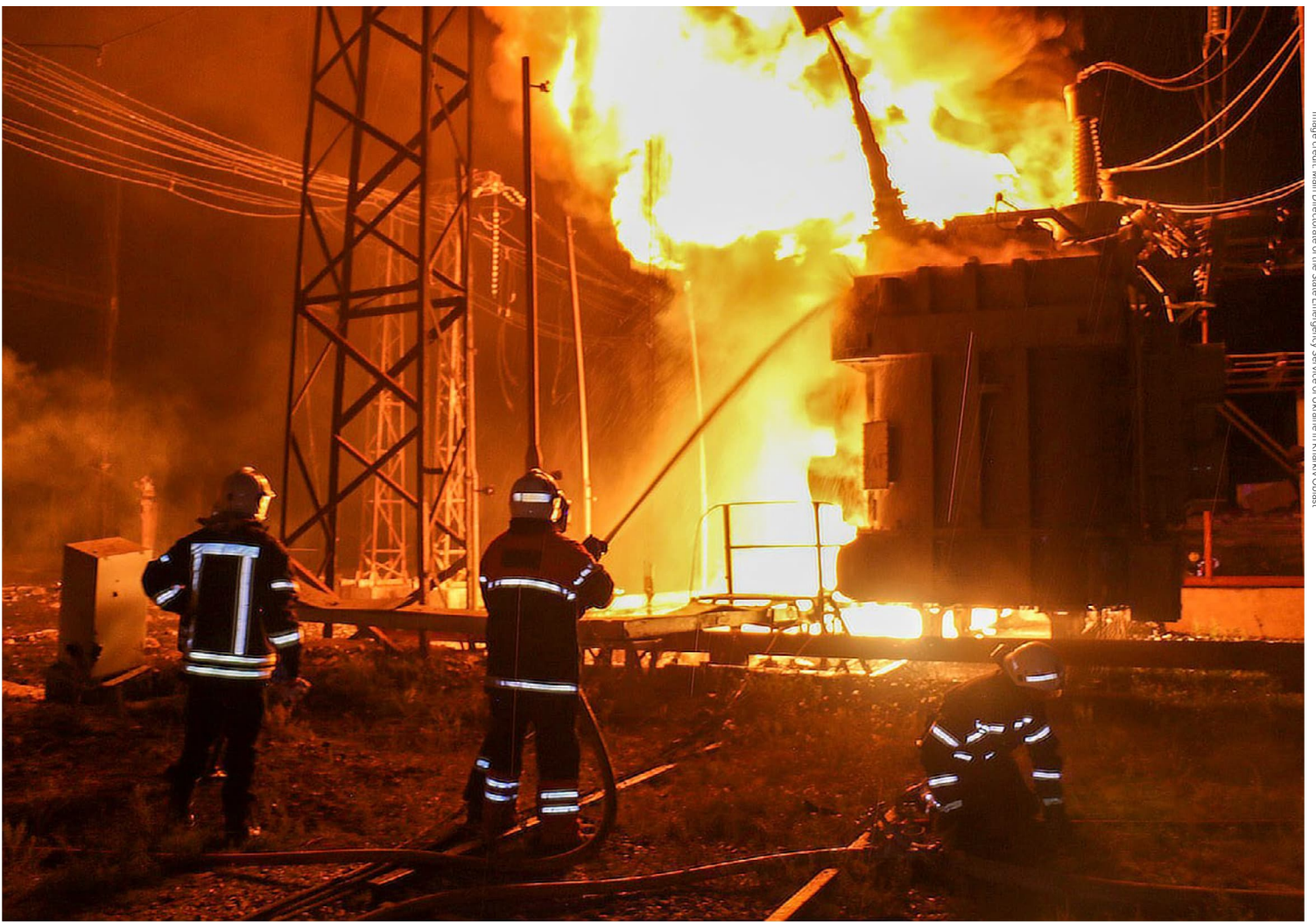
Fire at an energy infrastructure facility after Russian shelling
