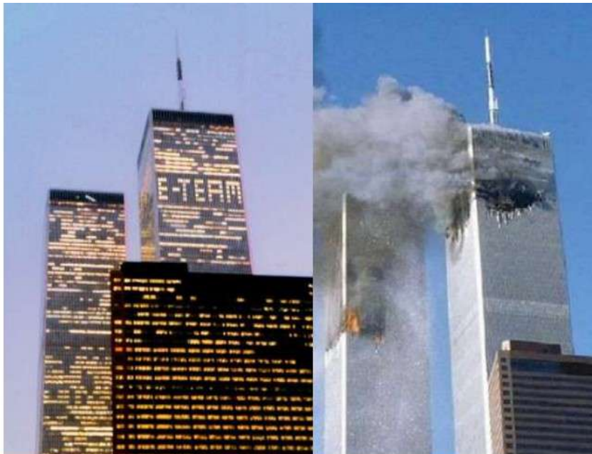
E-TEAM'S "127 LIGHTED WINDOWS" COMPARED TO DAMAGE ON 9/11
