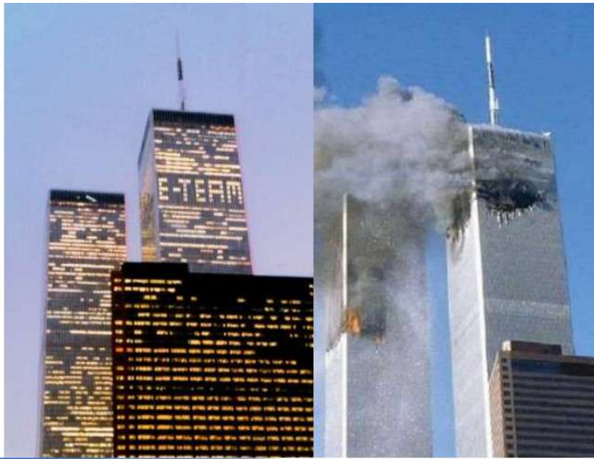
E-TEAM'S "127 LIGHTED WINDOWS" COMPARED TO DAMAGE ON 9/11
