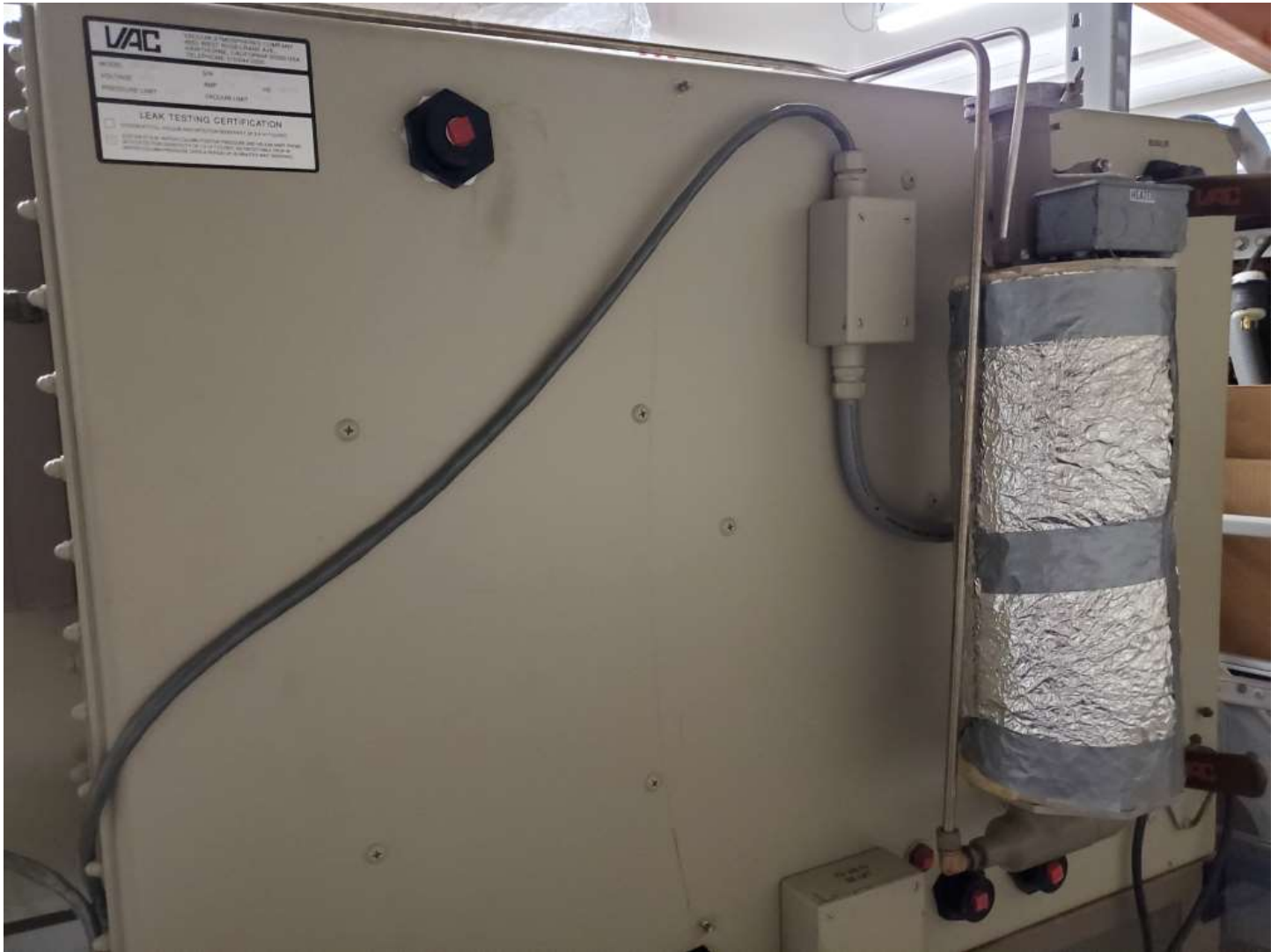
Purifier catalyst bed mounted on rear of glovebox
