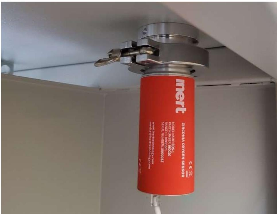
*Inert* zirconium oxide trace oxygen sensor. O<sub>2</sub> is level displayed on *Inert* control panel
