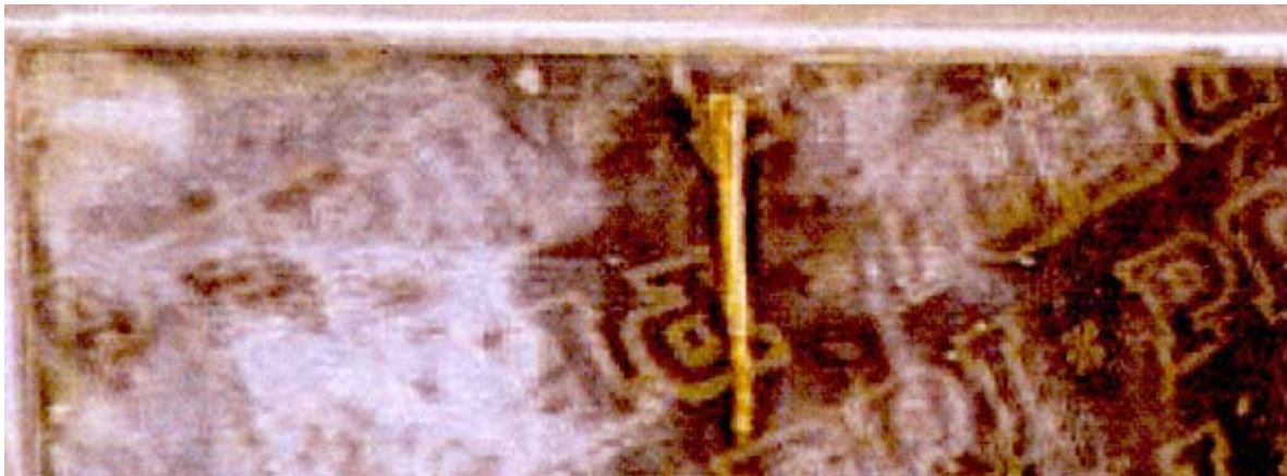
Photo 15: Non-permissible scratches in the formlining (depth > 1 mm)
