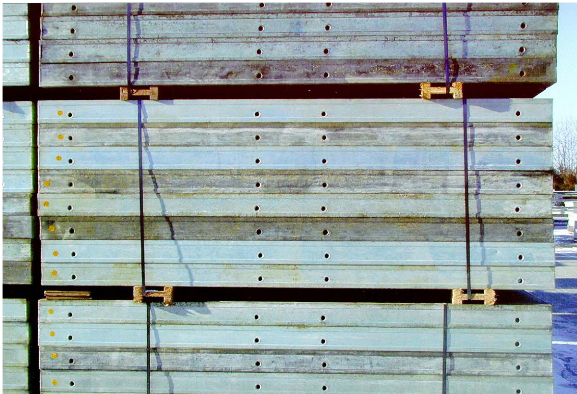
Photo 2: Example of required cleaning condition of the contact areas
