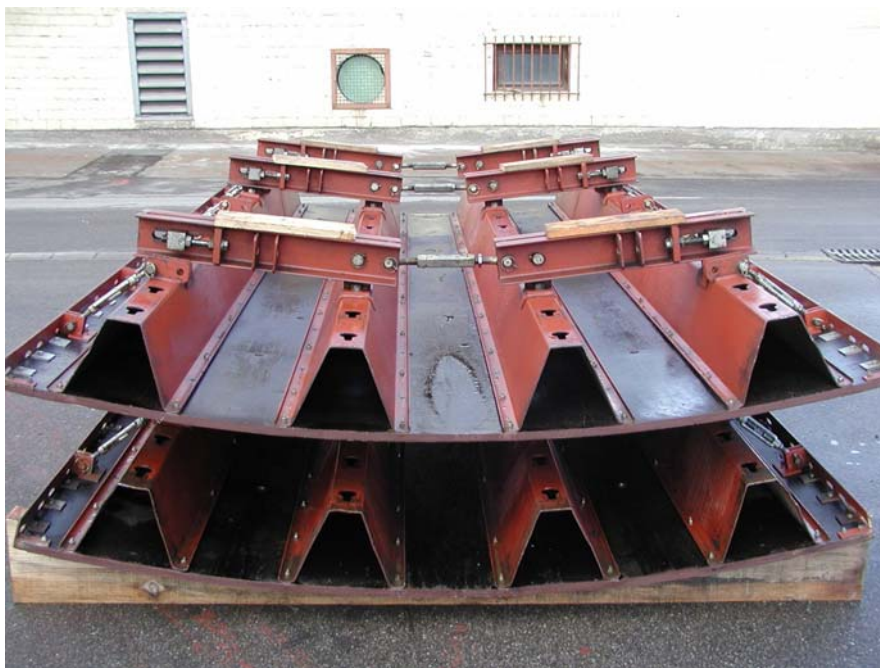
Photo 7: Use of timbers for stacking formwork panels
