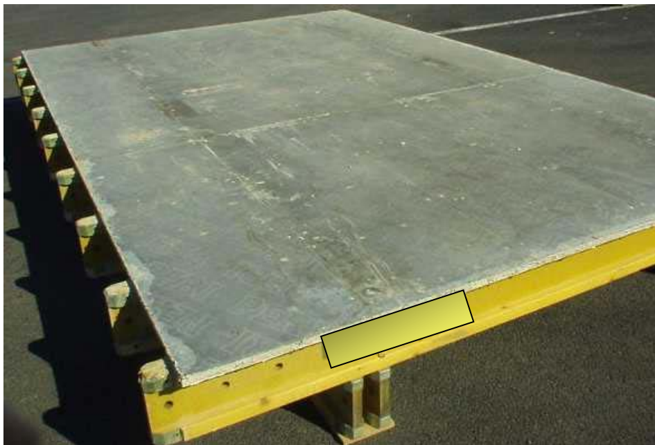
Photo 17: Permissible cleaning condition
