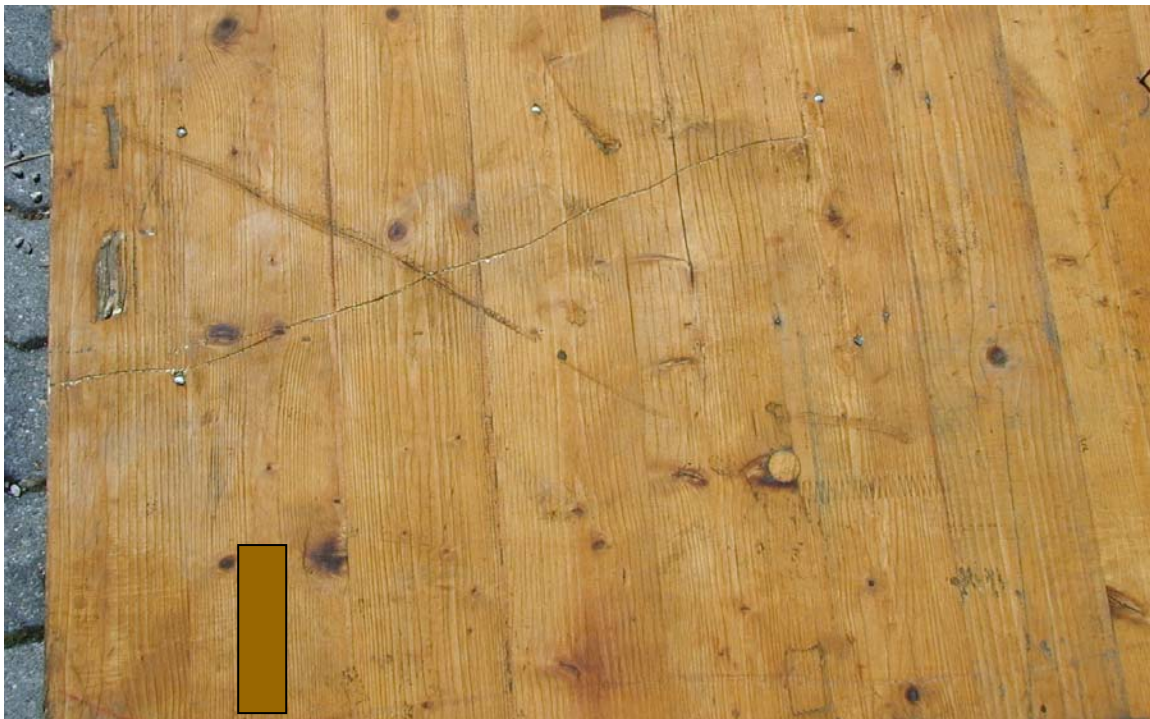
Photo 3: Permissible surface scratching
