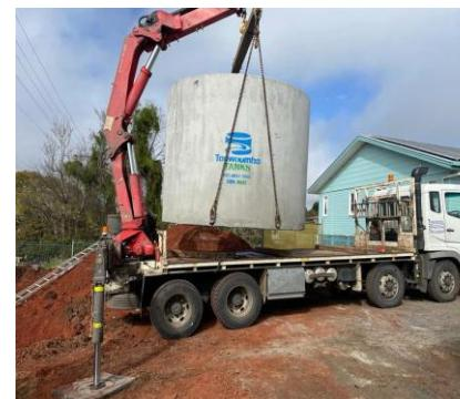
22,500 litres underground rainwater tank
