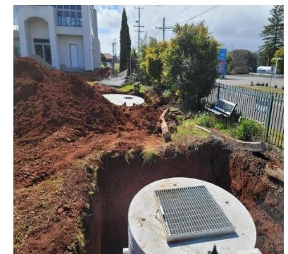
Manhole for stormwater management
