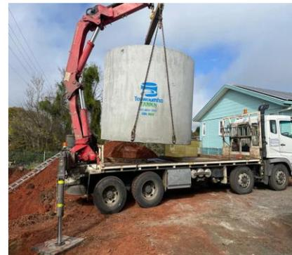
22,500 litres underground rainwater tank
