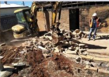
Rebuilding Start, Oct. 2018
