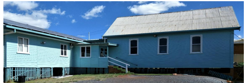
Newly painted front area of prayer hall
