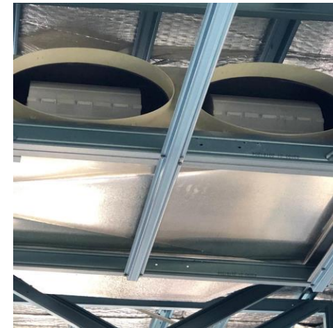
Photo: Second Stage work in progress
