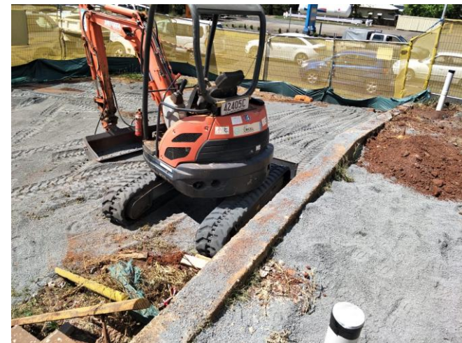
Completion of earth filling after connecting the new sewerage line.
