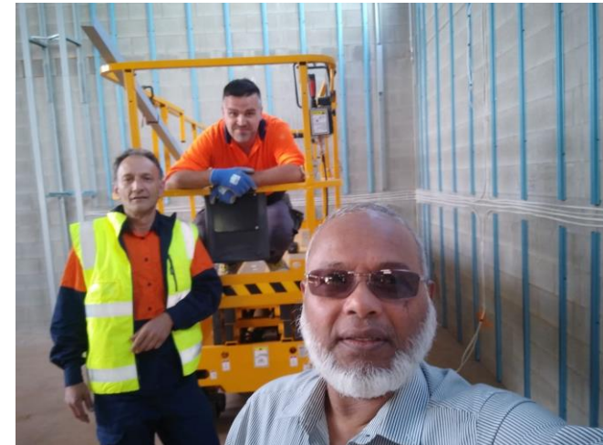
The builder working with the plasterer to fit the drop bolcet.
