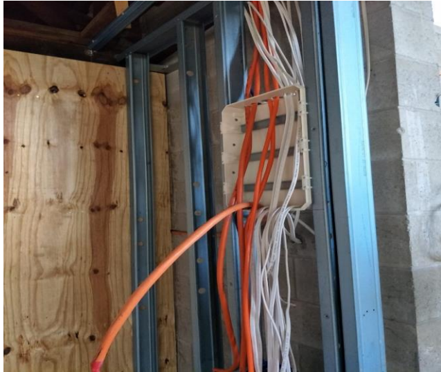
Connection of new switchboard to the main power line.
