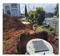
Manhole for stormwater management
