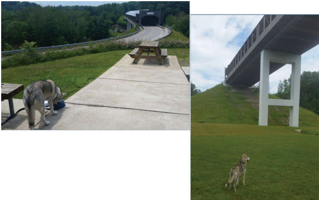
Above and below the Smolen-Gulf bridge
