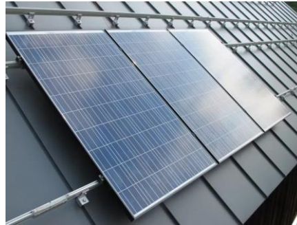
Solar PV panels over standing seam
