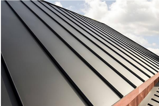
Standing seam roofs and concealed gutters
