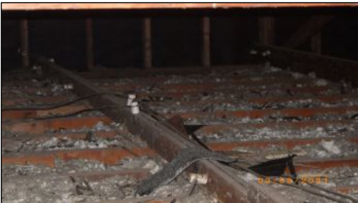
knob and tube wiring
