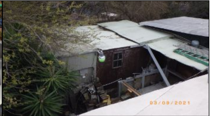
detached structures; bad condition
