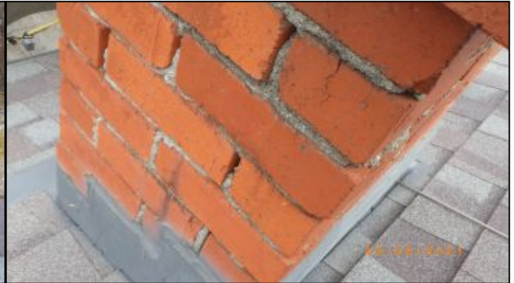
deteriorated mortar
