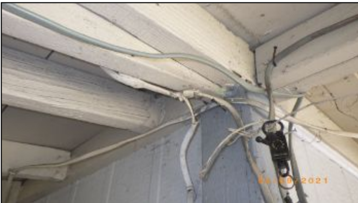
improper wiring
