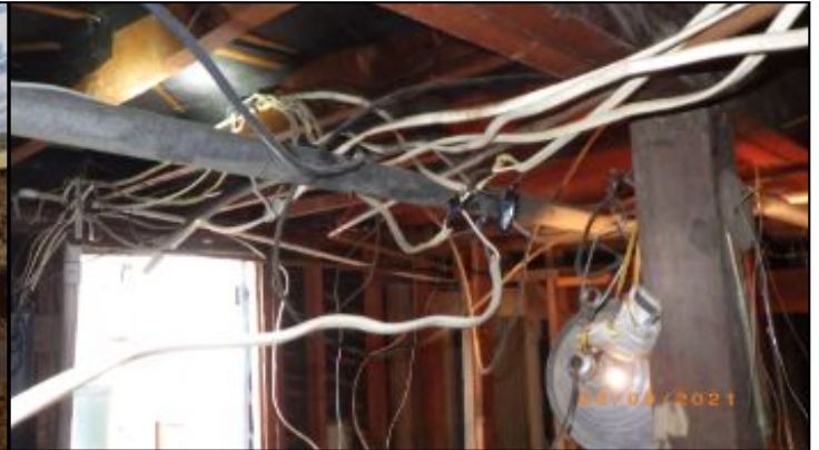
loose wires\improper wiring
