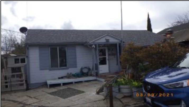
slope at front
