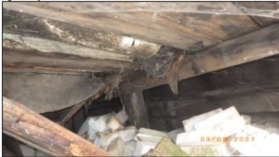
several aspects of outbuildings poor
