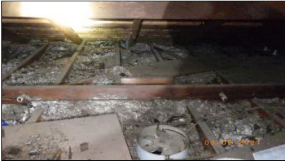
worn and heavy debris
