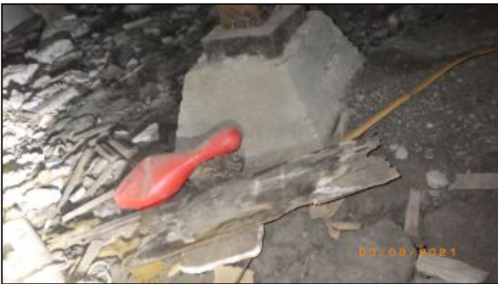
debris in crawlspace
