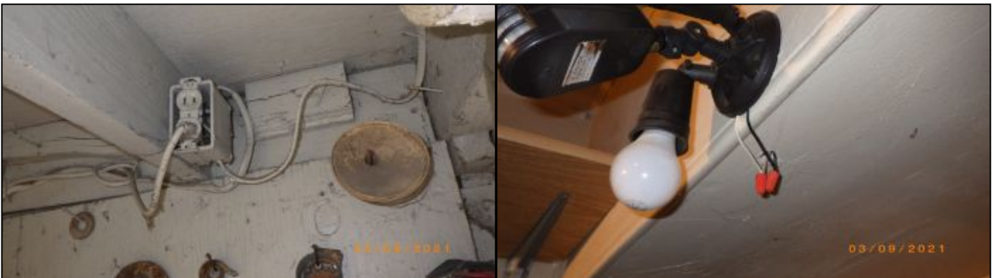
outlet missing cover
