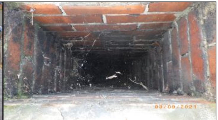
unlined masonry chimney
