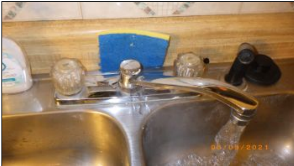
leak at kitchen sink
