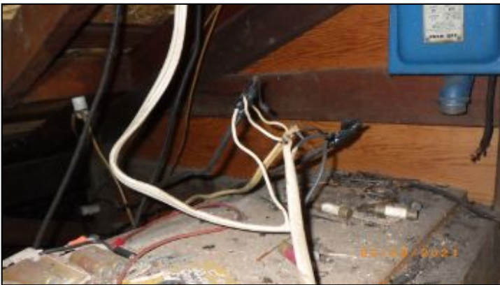
improper splices
