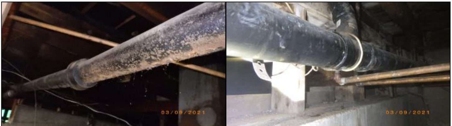
cast iron waste line
