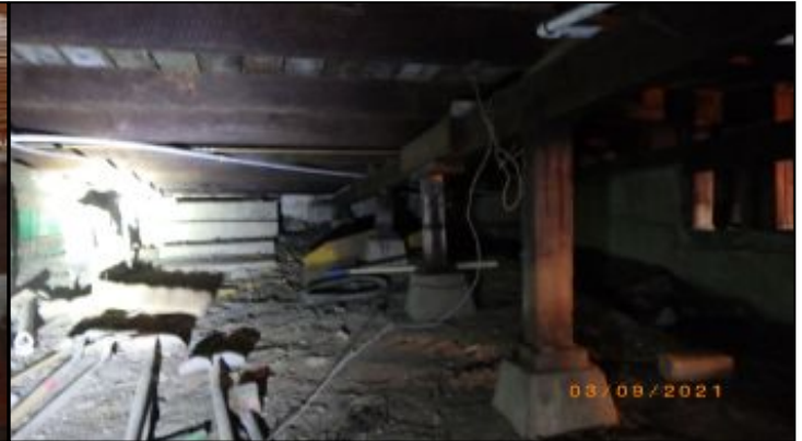
improper framing
