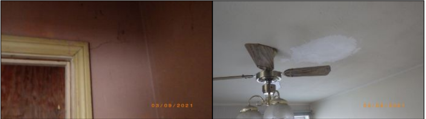
settlement cracks
