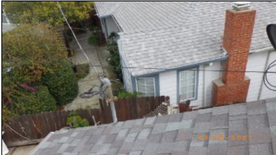
overhead service drop
