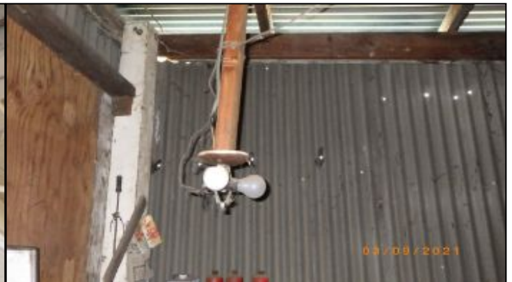
improper wiring
