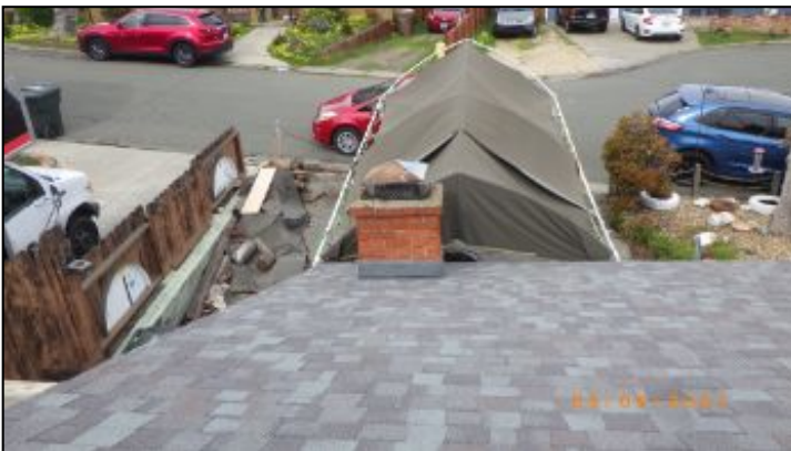
chimney too short
