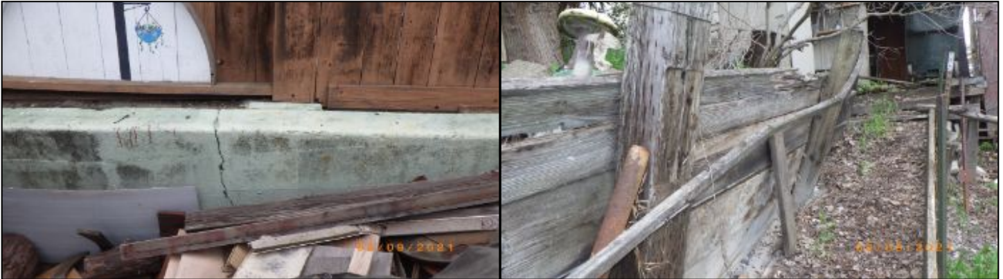
displacement visible at retaining wall
