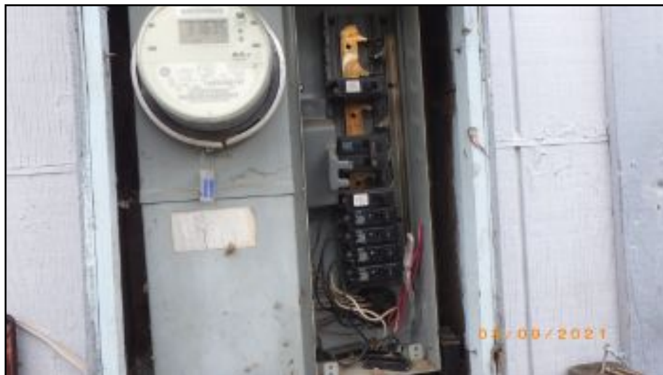
breakers not labeled; inner panel missing
