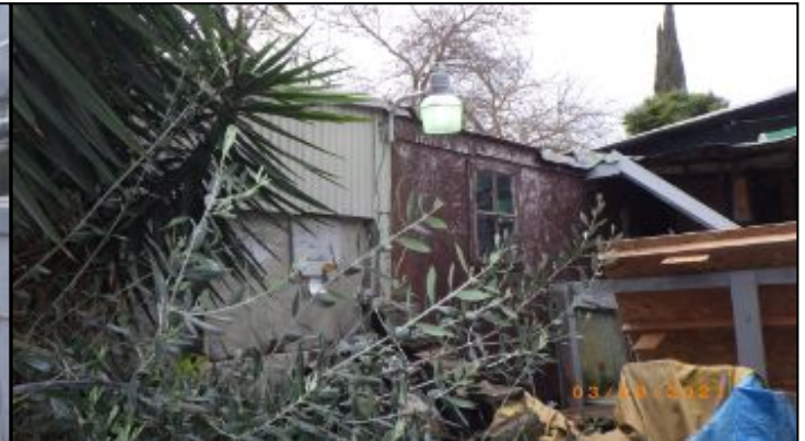
detached buildings not inspected, but in generally poor condition
