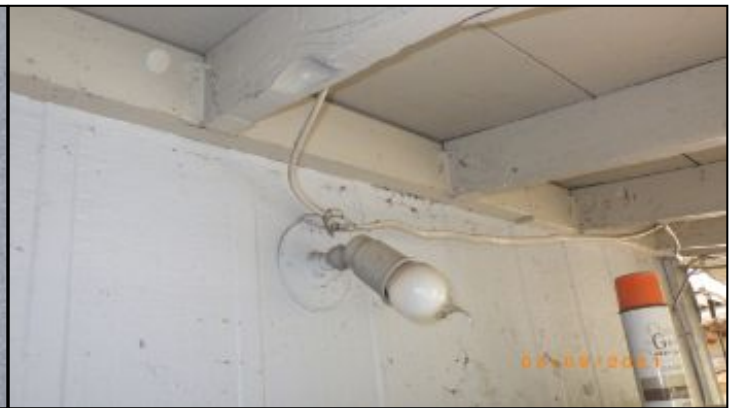
exposed cables/wire
