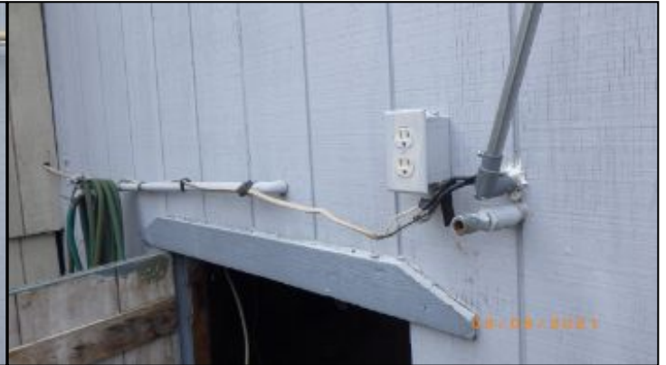
improper wiring
