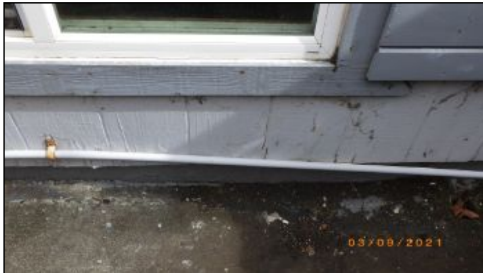
PVC distribution plumbing
