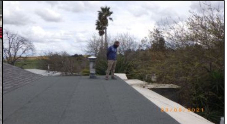
torch down section of roof
