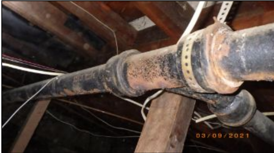
waste line rust cysts
