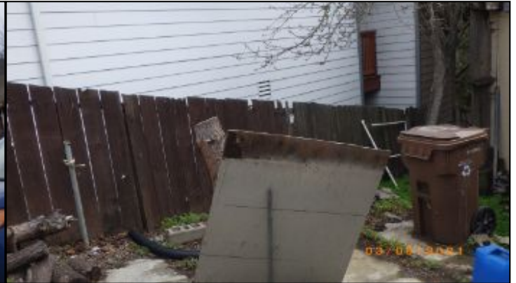
steep slope at the rear
