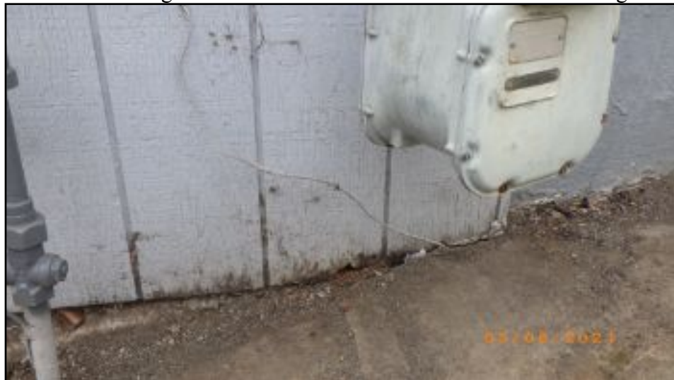
siding in contact with concrete
