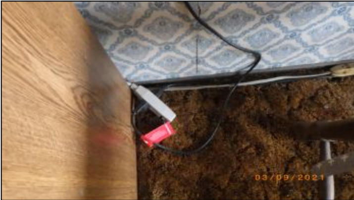
extension cords at interior
