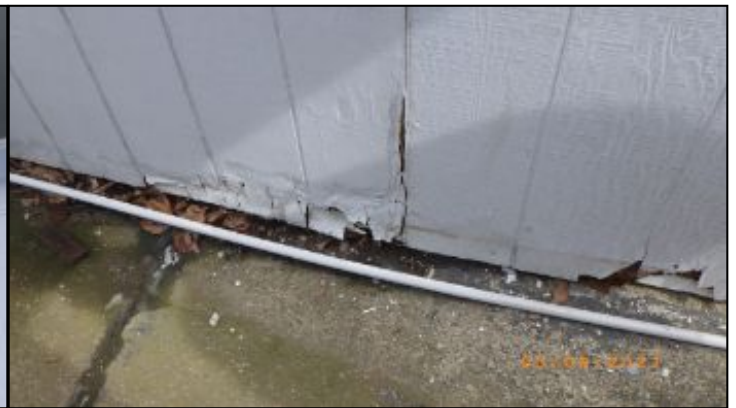
moisture damaged siding
