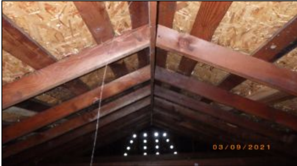
OSB over skip sheathing
