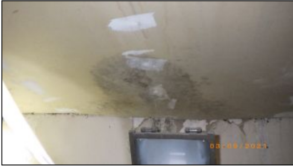
mold visible in laundry room
