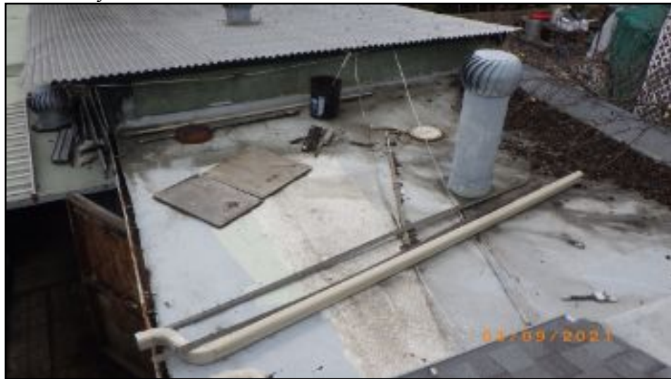
debris on roof
