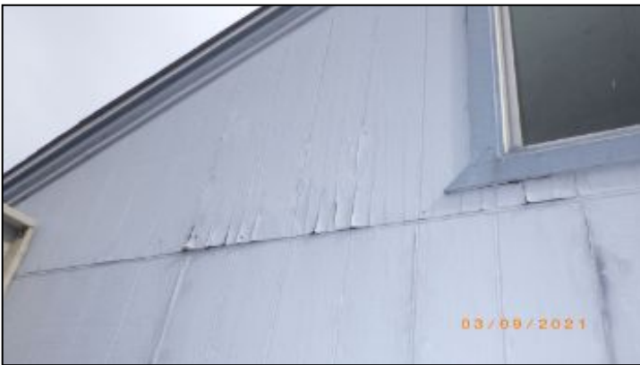
delaminated siding
