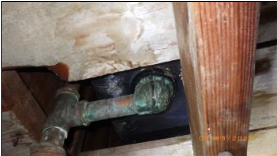
drain leak
