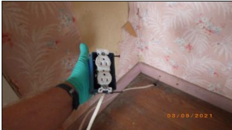
several aspects improper
