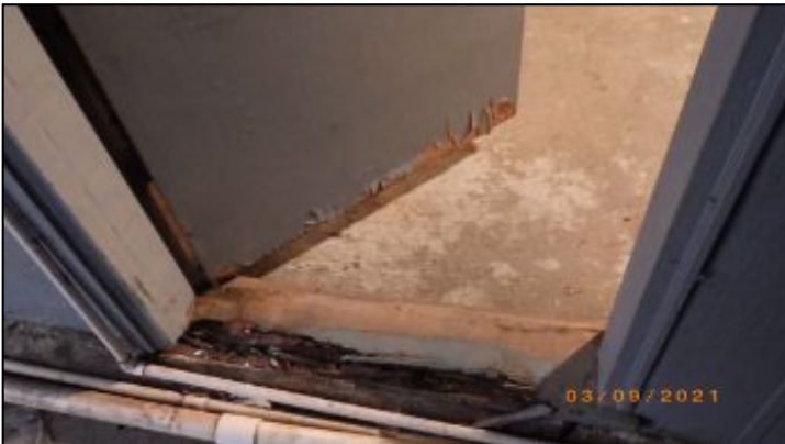
moisture damaged door
