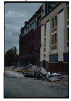
The building on the southeast corner of Sixth and Bluxome streets was a four-story structure and the fourth floor wall peeled away from the building during the earthquake and showered the street below with tons of bricks. Five people were killed, crushed in their automobiles or while walking upon the sidewalk.
