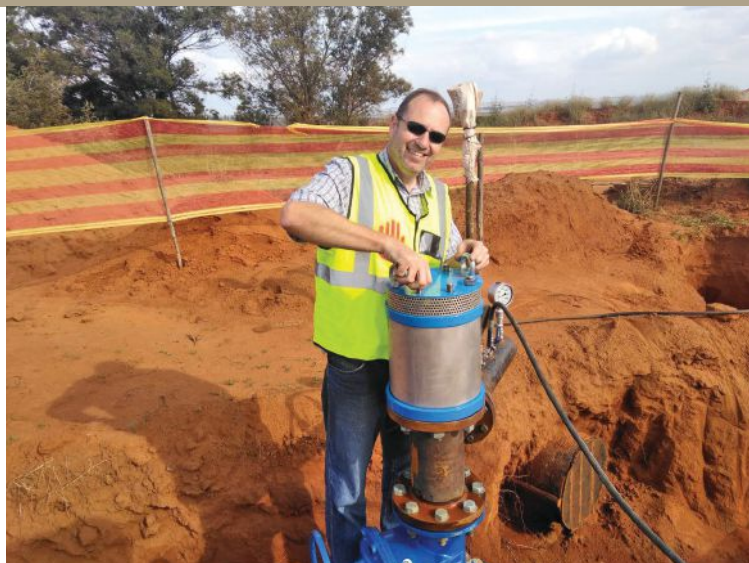
Dave Dolman installing an advanced air valve.
