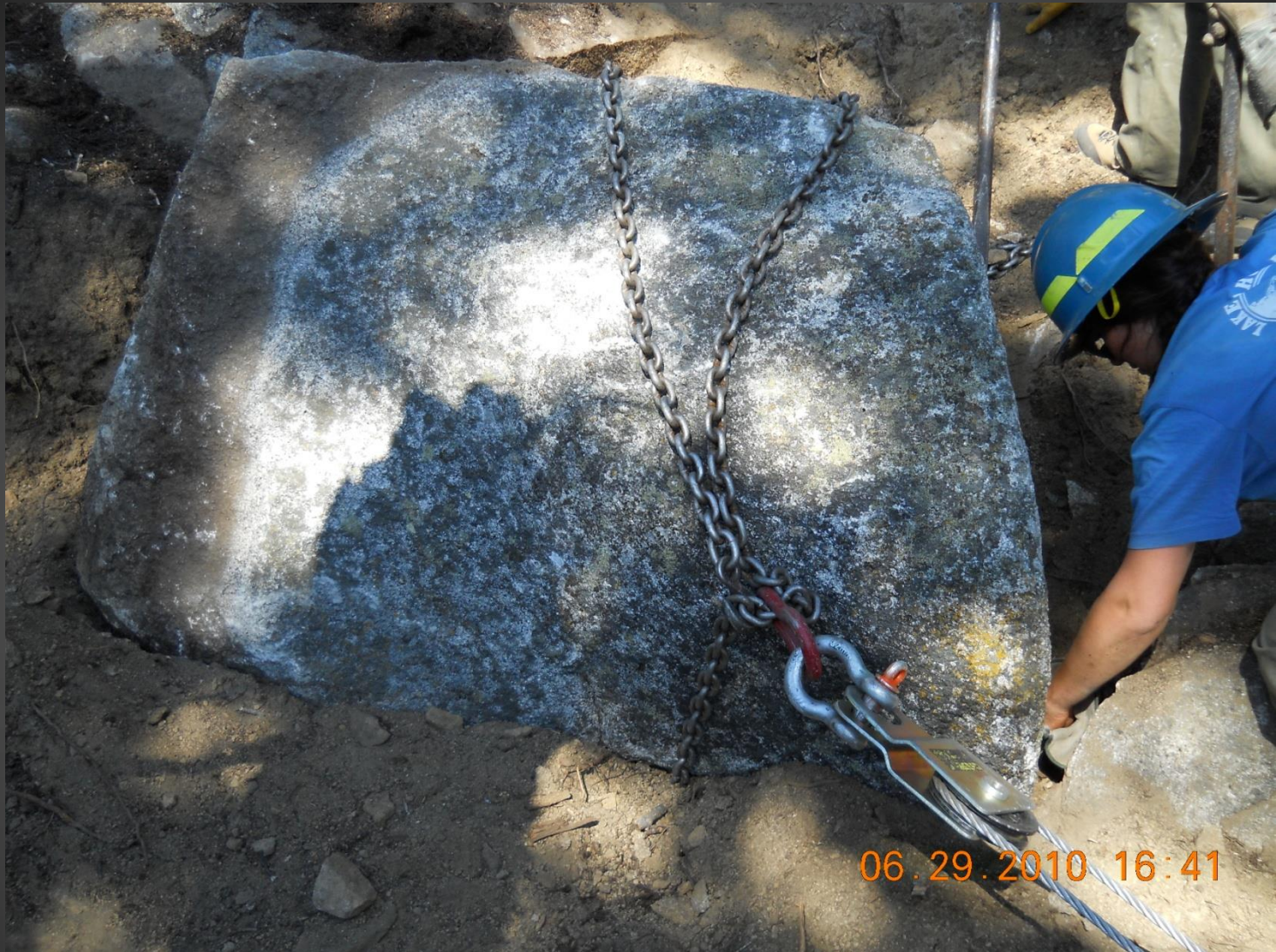
Chain double-wrapped around boulder, keyhole link to connect to chain, shackle connecting keyhole link to block, block setup as 2:1
