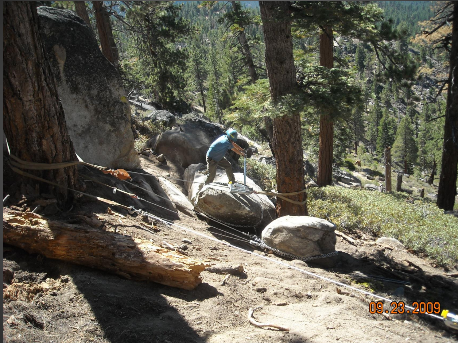
Griphoist #1 (center of photo): directional change only Griphoist #2 (far right): 2:1 MA with additional block as a directional
