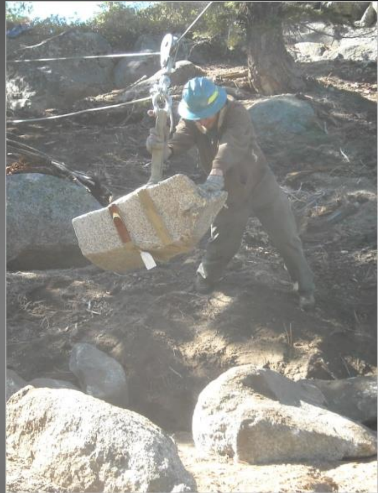
Sling in choker orientation
