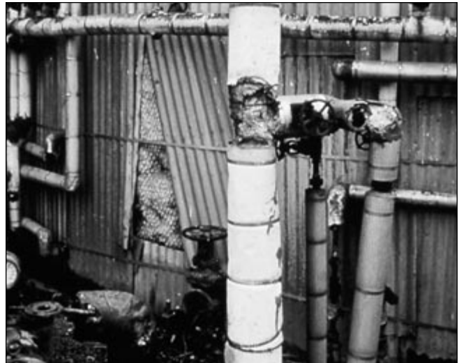
Loose fill insulation
