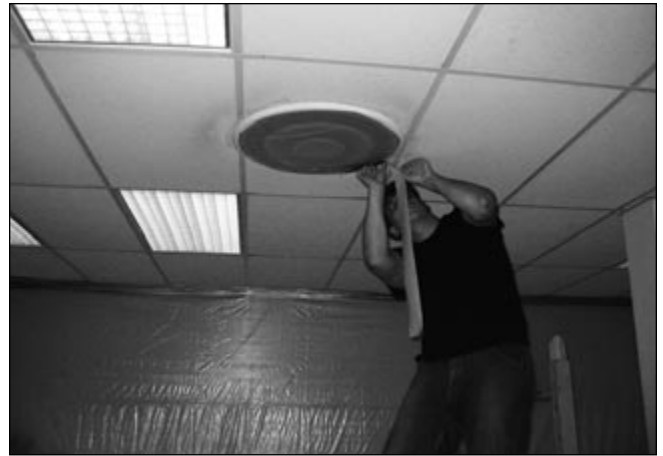
Sealing the ventilation system
