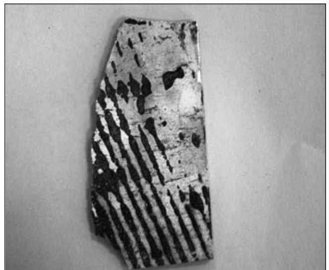
Vinyl asbestos flooring
