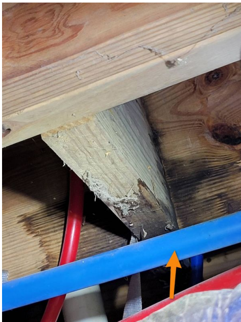
Multiple locations. Previous water damage
