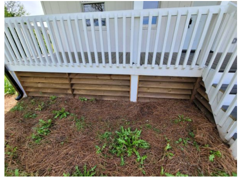
Underneath front porch
