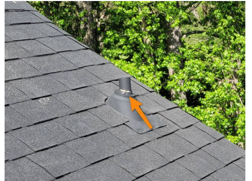
Separation of another boot (multiple locations)
