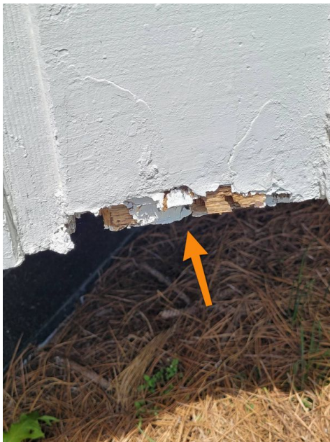
Left around kitchen bay window. Multiple locations
