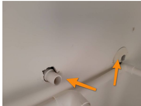
Abandoned old pipe system
