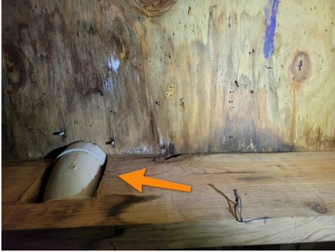
Multiple joists cut for plumbing
