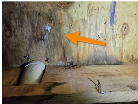
Multiple locations. Previous water damage
