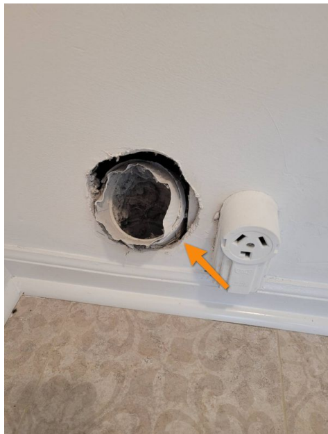
Dryer vent recessed and not sealed off to crawl
