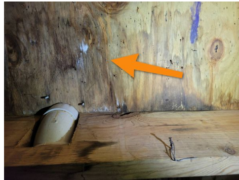
Multiple locations. Previous water damage
