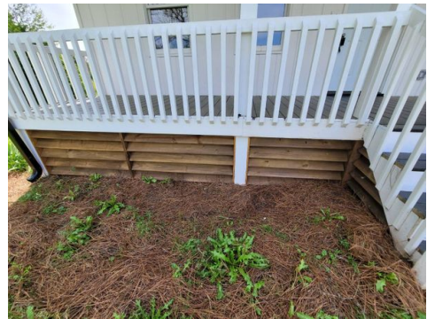
Underneath front porch
