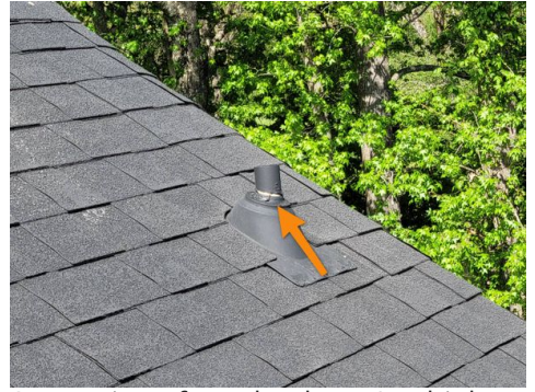
Separation of another boot (multiple locations)
