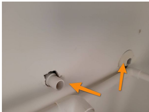
Abandoned old pipe system
