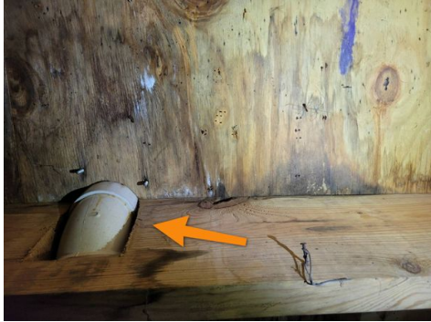
Multiple joists cut for plumbing
