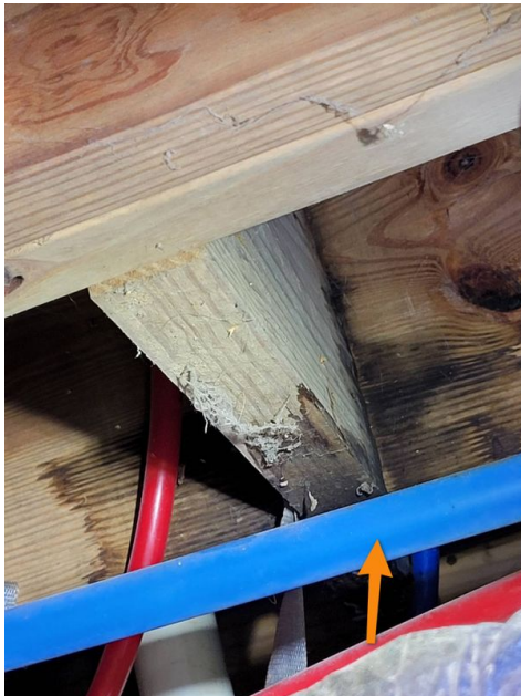
Multiple locations. Previous water damage
