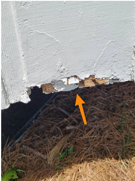
Left around kitchen bay window. Multiple locations
