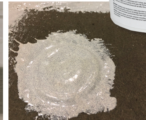
Acclaim® FSG applied by chip brush over fastener head, plate and seam on an impact resistant cover board system prior to coatings application.
