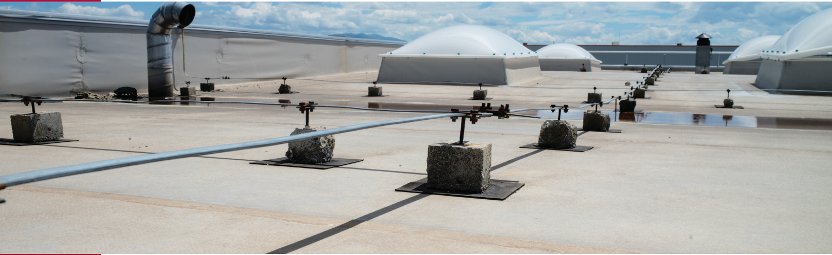
Acclaim Pond B Gone applied in a low scupper area over an aged acrylic roof coating prior to application acrylic recoating system.
