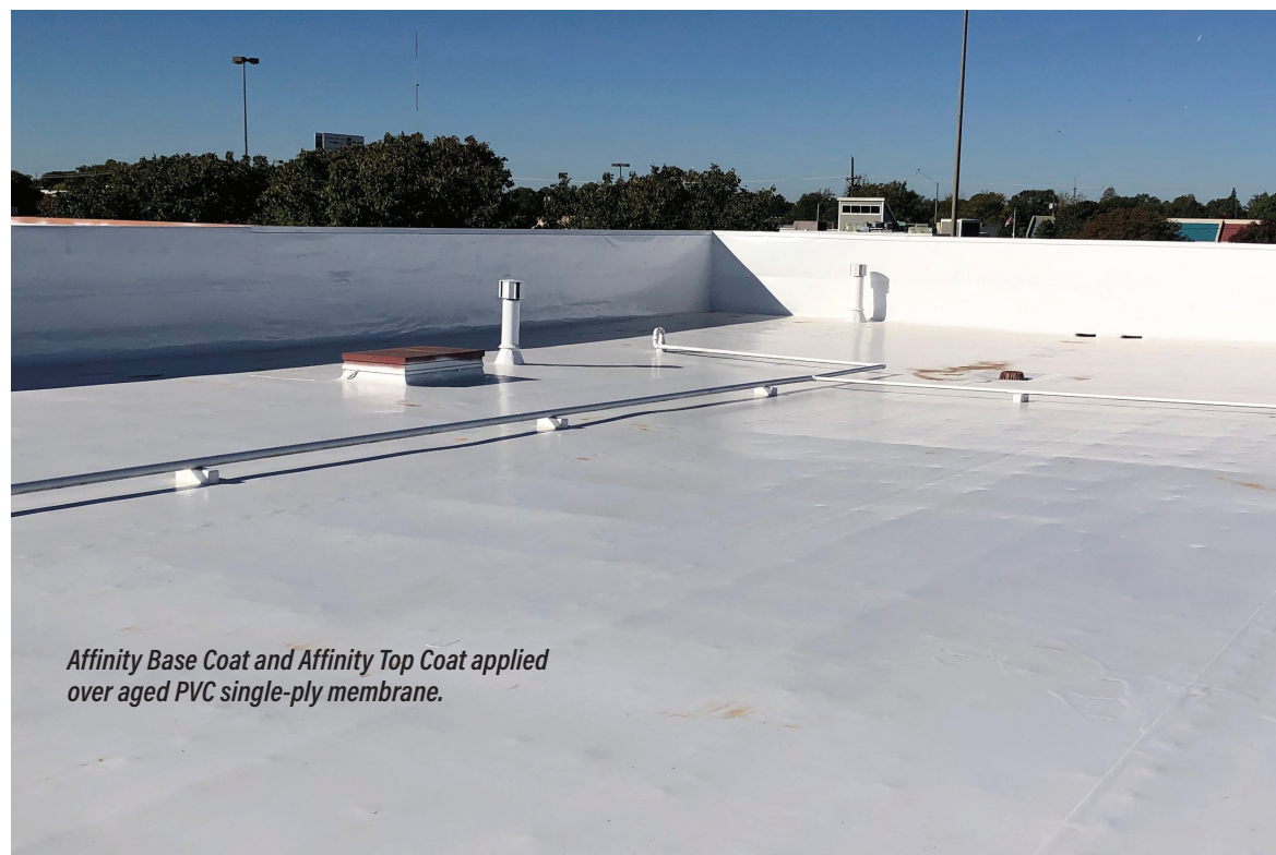
Affinity Base Coat applied over aged PVC single-ply membrane.
