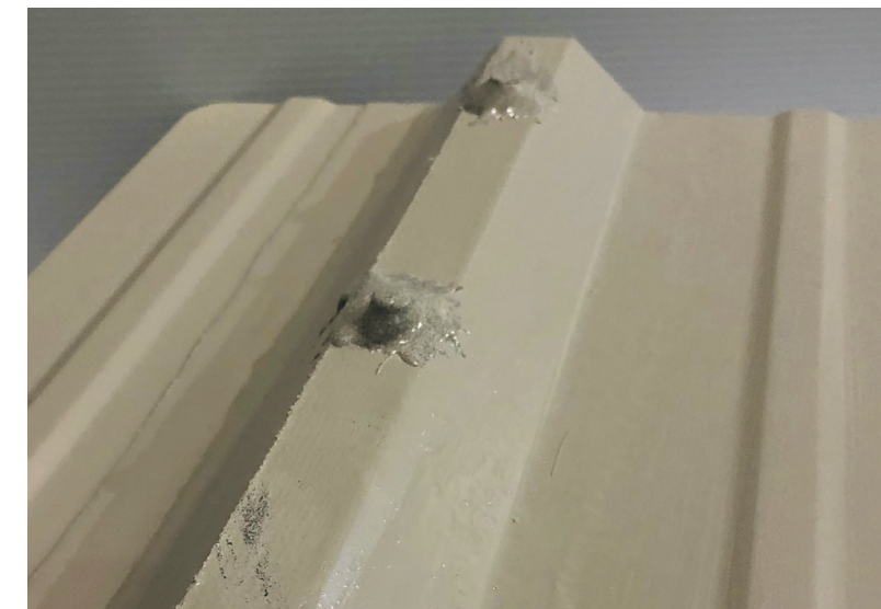
Acclaim® FSG applied by chip brush over fastener head, plate and seam on an impact resistant cover board system prior to coatings application.
