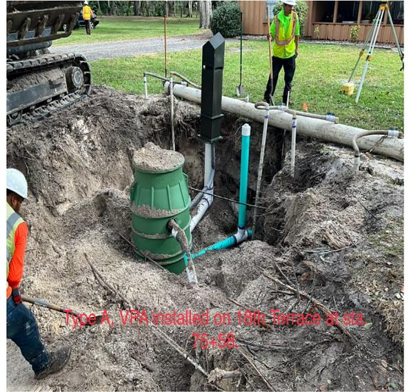
Type A, VPA installed on 18th Terrace at sta. 75+50
