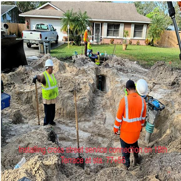
Installing cross street service connection on 18th Terrace at Sta. 77+56
