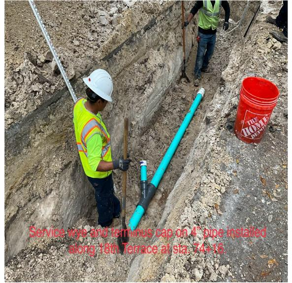
Service eye and terminal cap on 4" pipe installed along 18th Terrace at sta. 74+16
