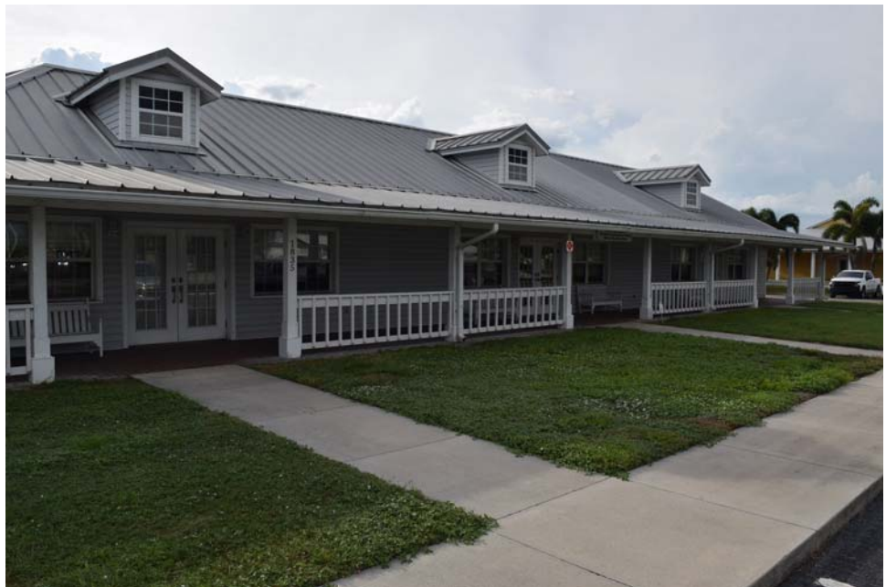
View of eastern portion of subject building.
