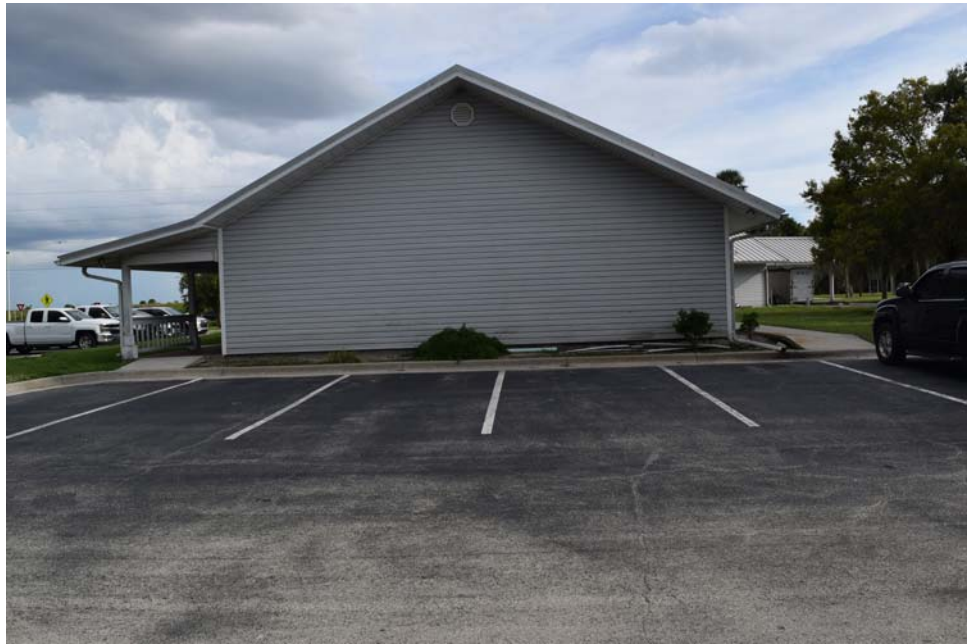
View of north end of subject building from parking lot.
