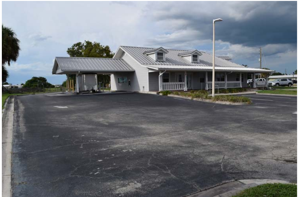
View of southern portion of subject building from south boundary.
