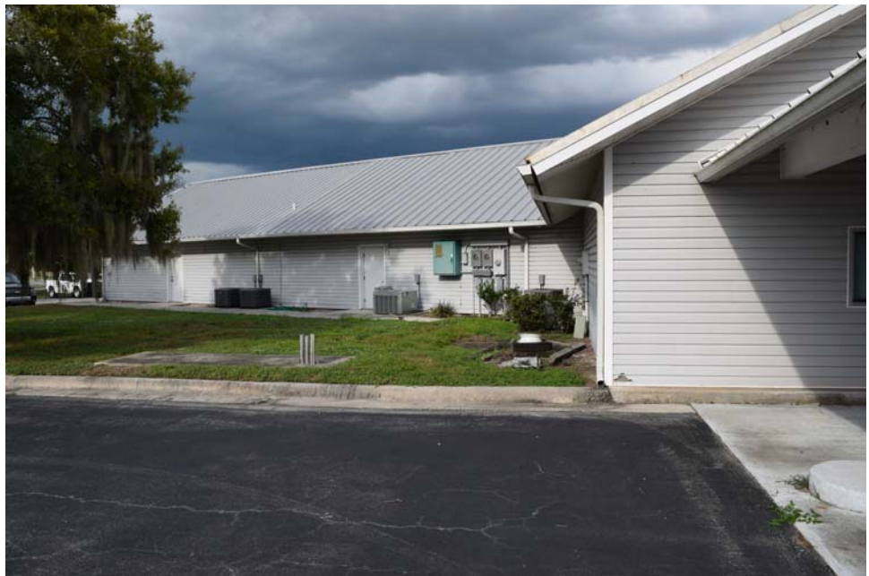
View of rear of subject building from drive-thru area.
