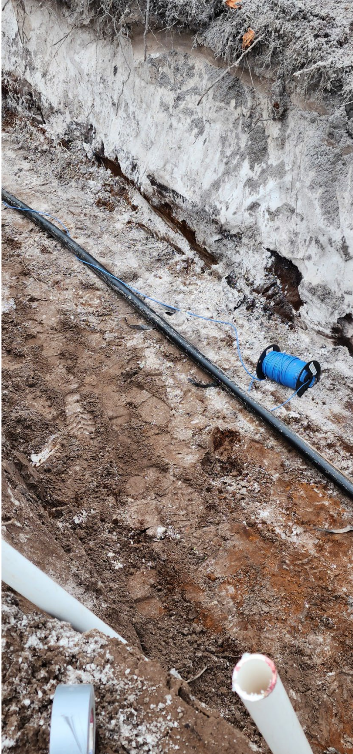
8 - Water Service with Locator Wire
