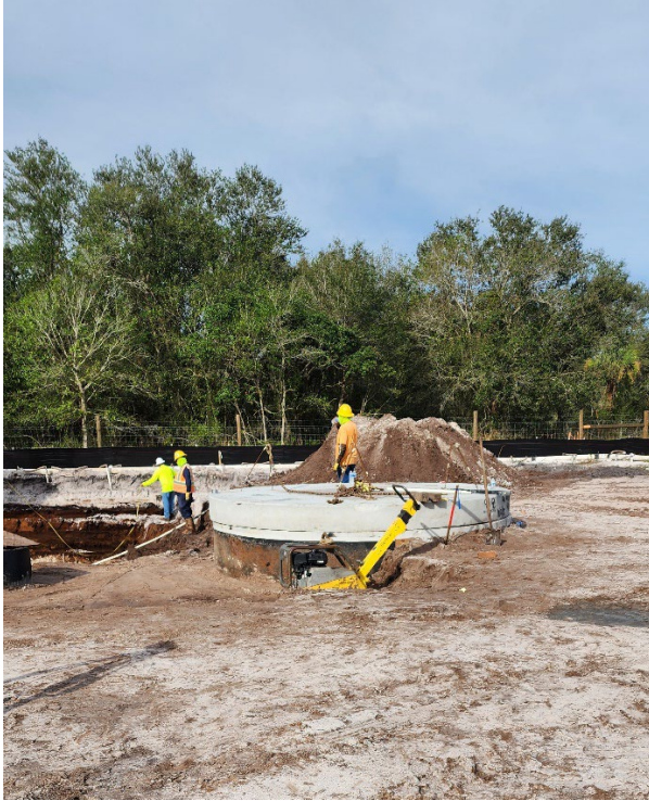
1 – Compacting around Wet Well
