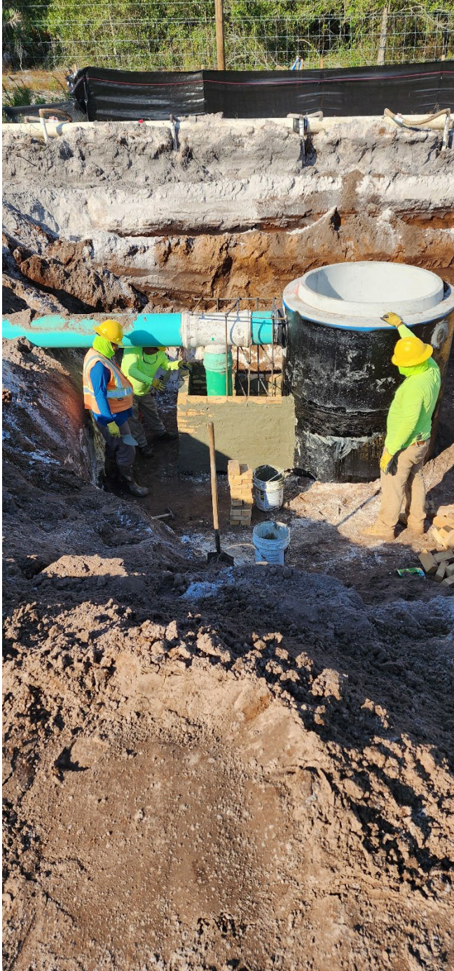
5 - Outside Drop (Force Main into Manhole 3)
