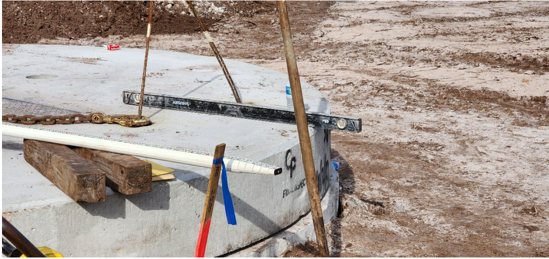
3 – Leveling Wet Well
