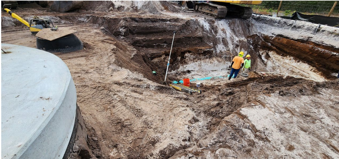
4 – Gravity Sewer – Manhole 1 to Manhole 2
