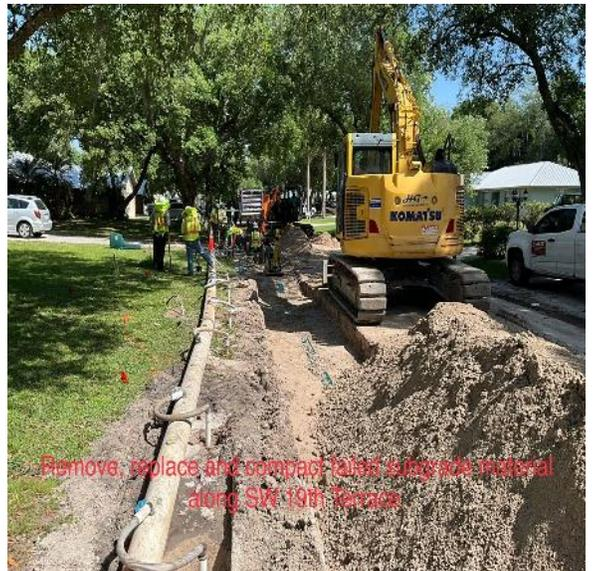
Remove, replace and compact failed subgrade material along SW 19th Terrace
