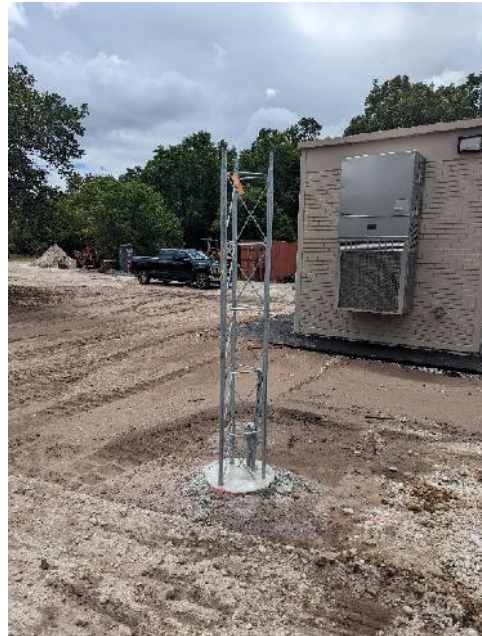
3 – SCADA Antenna (Partially installed)
