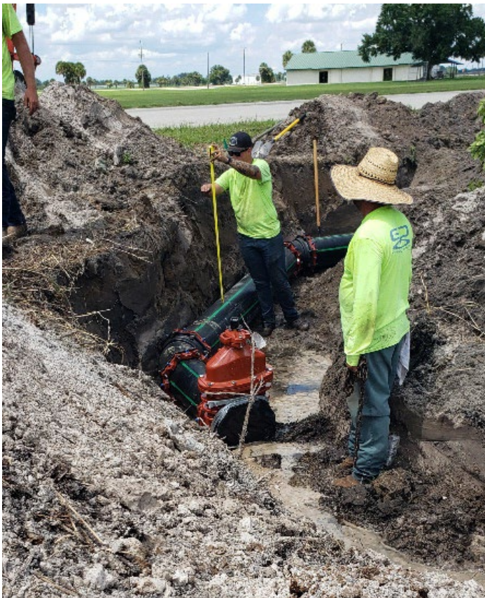
8 - Setting Valve and Fitting (Near Hall Property)
