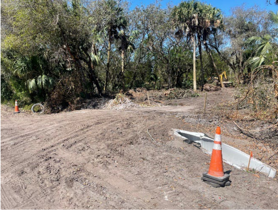
1 - Driveway Culvert, MPS Site
