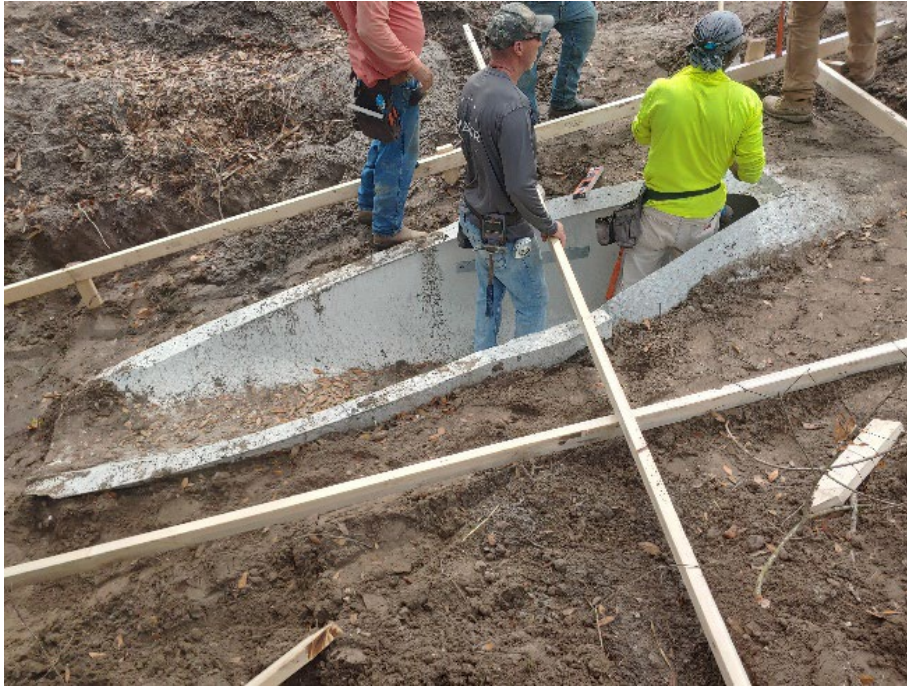
3 - Concrete Forms for M.E.S., MPS Site
