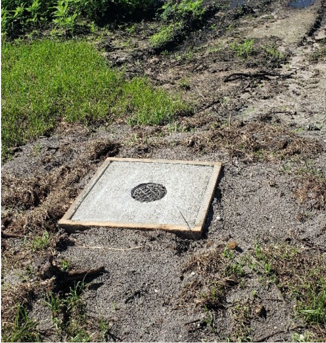
13 - Valve Box / Pad (Typical)
