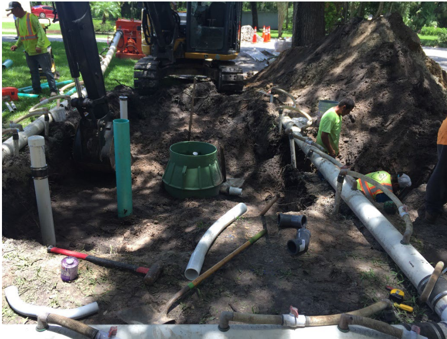
3 – Dewatering and Vac Pit Installation
