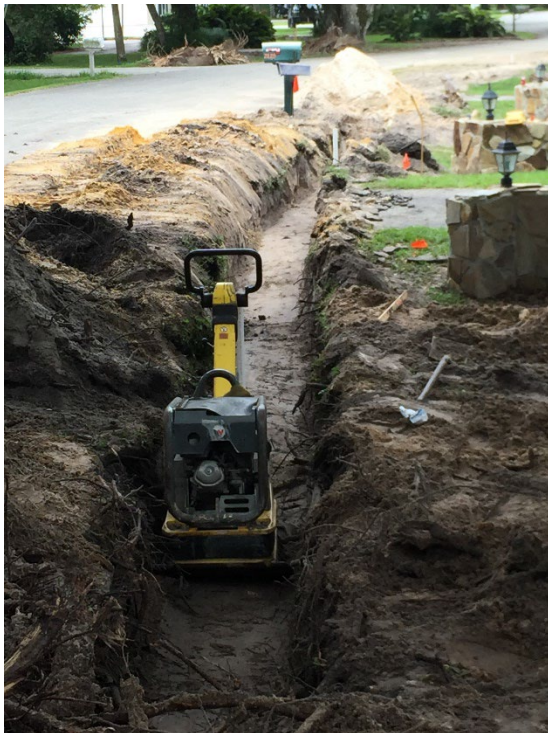
2 – Trenching, Backfill Compaction
