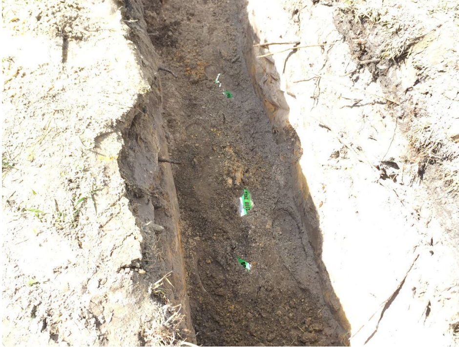
1 – Pipe Trench and Locator Tape
