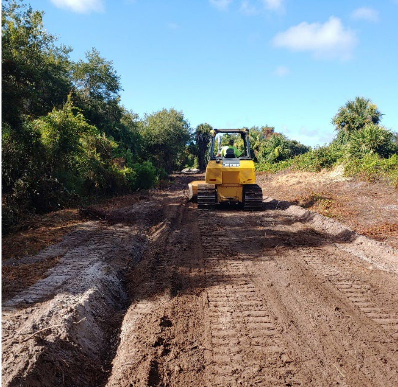
11 - Trench Compaction (School Board Easement)
