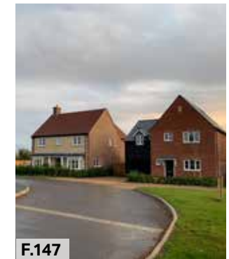
F.147 Figure 147: Unsympathetic roofline
