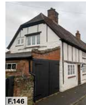
F.146 Figure 146: Halfhipped end at 50 degree
