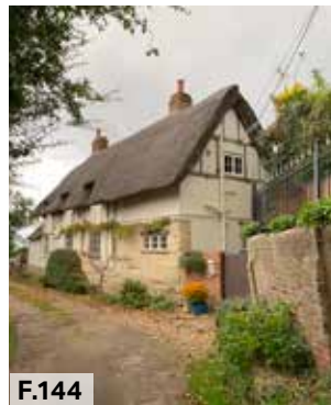
F.144 Figure 144: Full gables end at 55 degree
