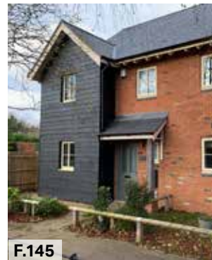
F.145 Figure 145: Full gables end at 45 degree
