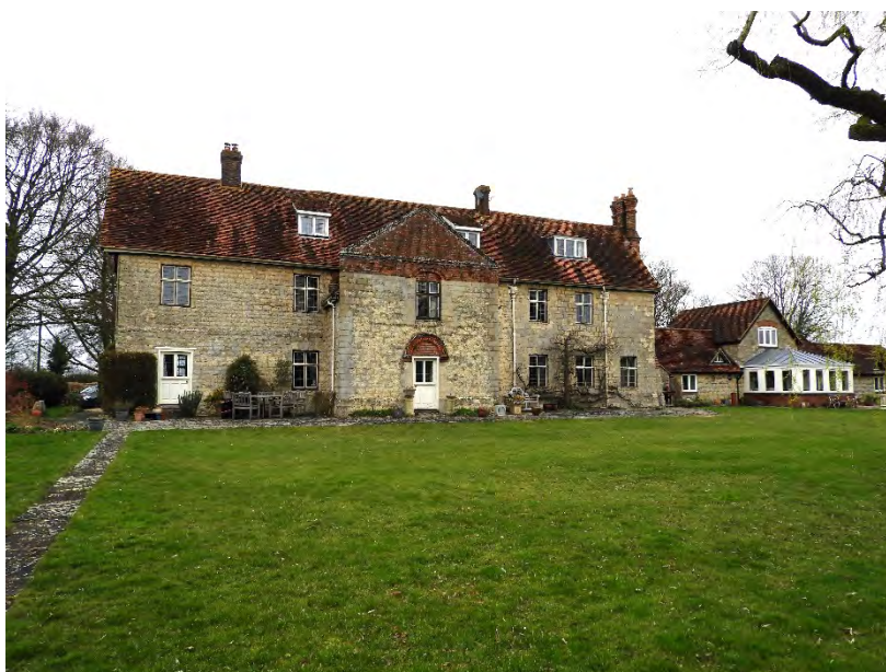
South (front) elevation of Kempson House
